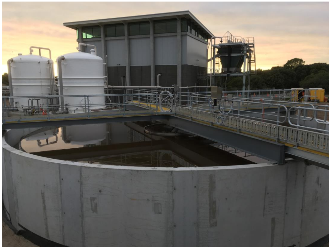
Photograph 5: PFTs, Dewatering Building and Loadout Silo
