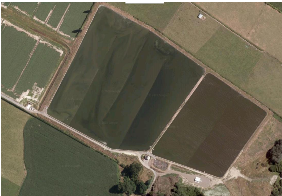
Figure 1: Matamata Wastewater Treatment Facility
