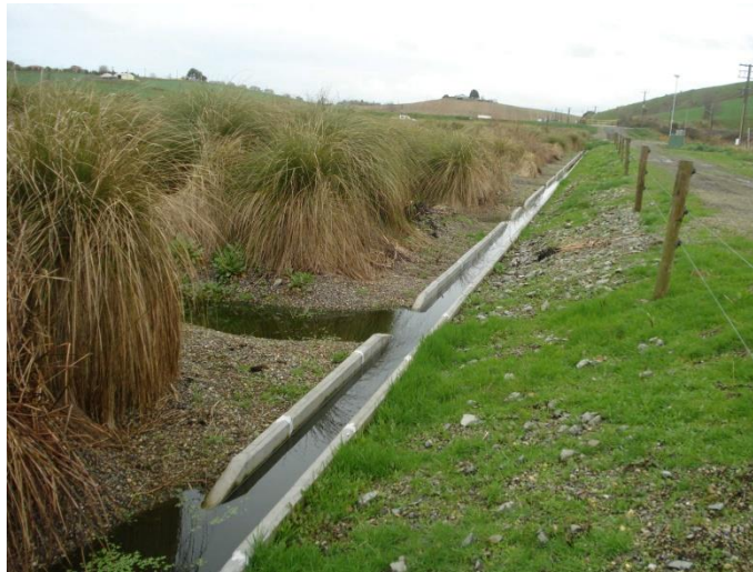
Gravel-bed Outlet Channel
