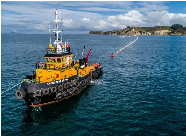
Figure 18: Pipe String 2 being pulled into tension
