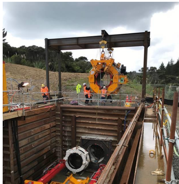
Figure 9: 750 tonne Thruster weighting 36 tonnes lifted with custom gantry
