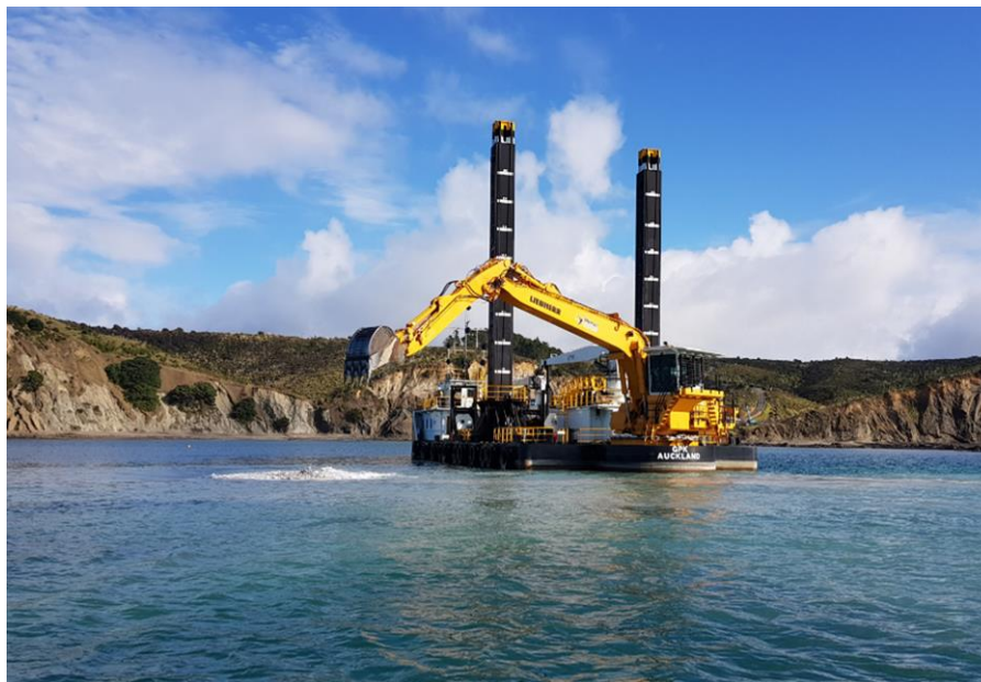
Figure 11: Herons Dredge, GPK on site excavating the transition pit
