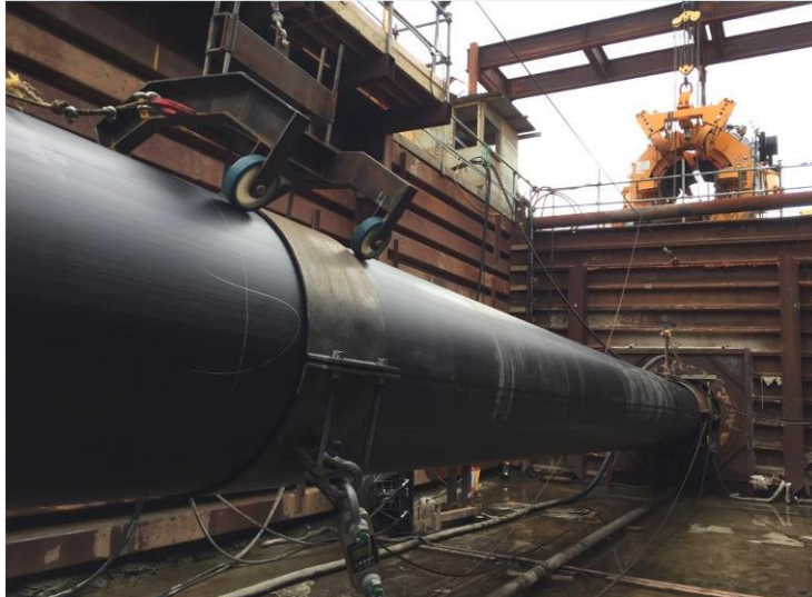
Figure 22: HDPE Liner Installation
