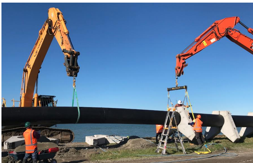
Figure 15: Installation of the Ballast Blocks
