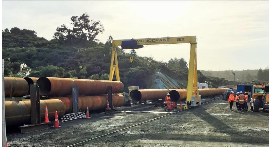
Figure 8: Welding bed with two pipe strings fabricated
