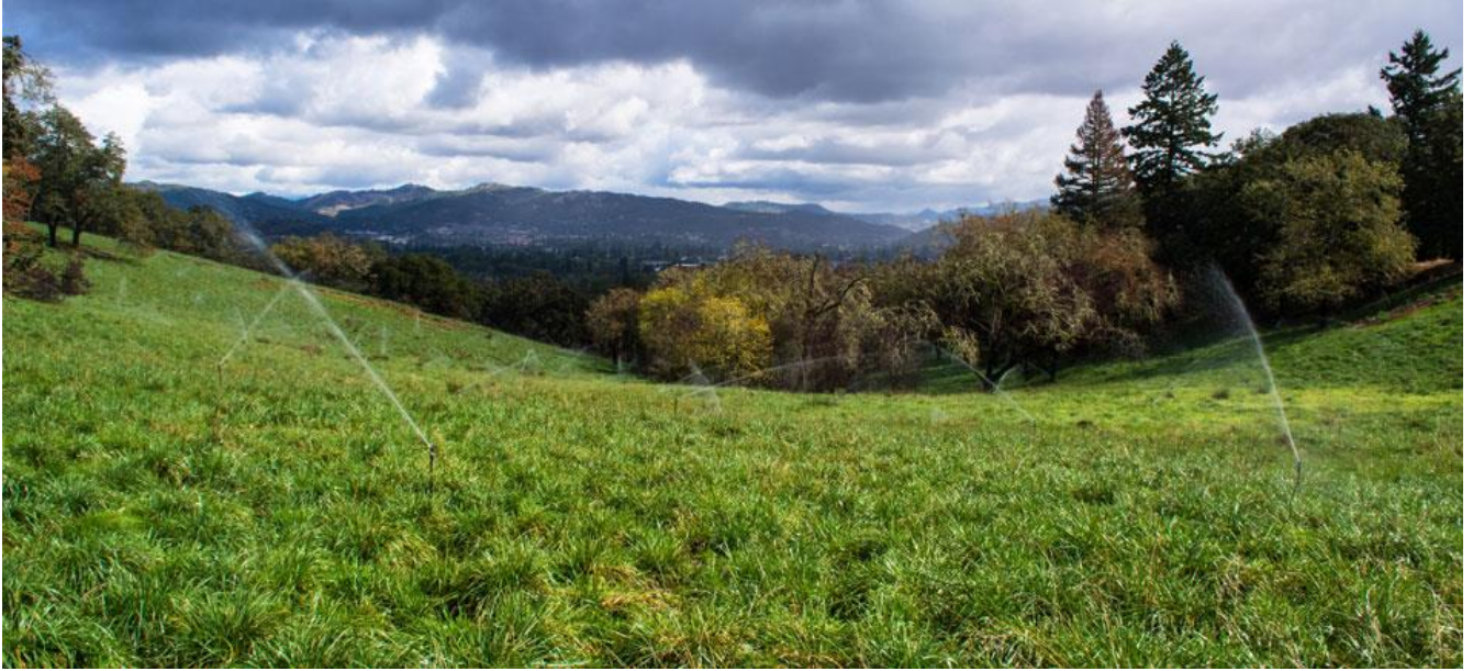
Figure 3. Land application system in Roseburg, Oregon, USA. Flow to this system is 13 MLD of advanced secondary effluent on 137 ha. The system is designed for phosphorus removal during dry weather. The irrigation plan keeps the soil permanently wet. Year-round discharge to land would be possible if irrigation were subsurface drip, but a larger area might be necessary for this hilly terrain. It is expected that in the 50-year expected lifespan of this system Roseburg urban development will expand around this area.
