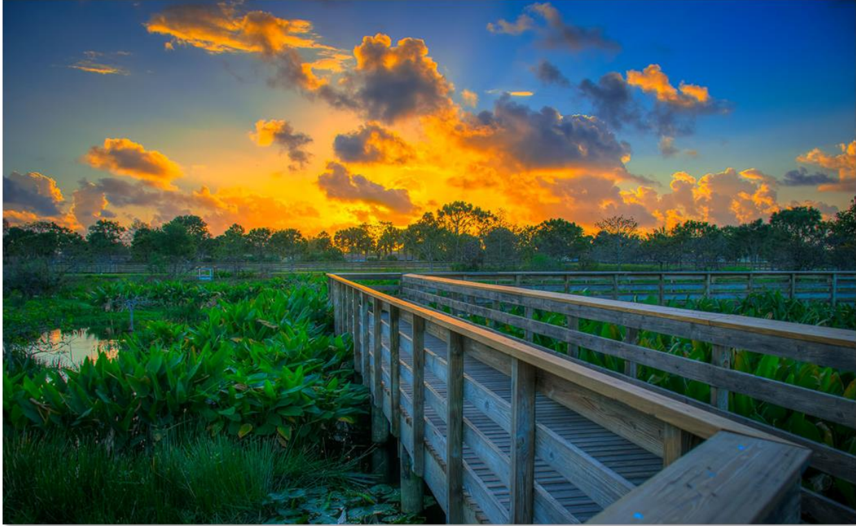
Figure 2. Wakodahatchee wetland in Palm Beach County, Florida, USA. The wetland takes approximately 19 MLD of secondary effluent and infiltrates it to groundwater in 18 ha of wetlands. There are approximately 1.2 km of boardwalks through the wetland that the public enjoys daily. The wetland is surrounded by urban development and is a top bird-watching area in Florida.
