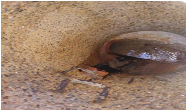
Exposed aggregate before relining
