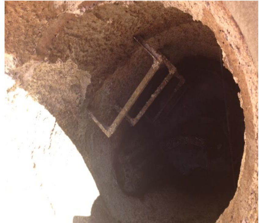
Manhole condition to prior to relining
