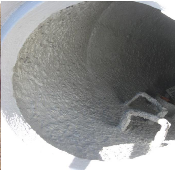
Figure 15: Manhole relined
