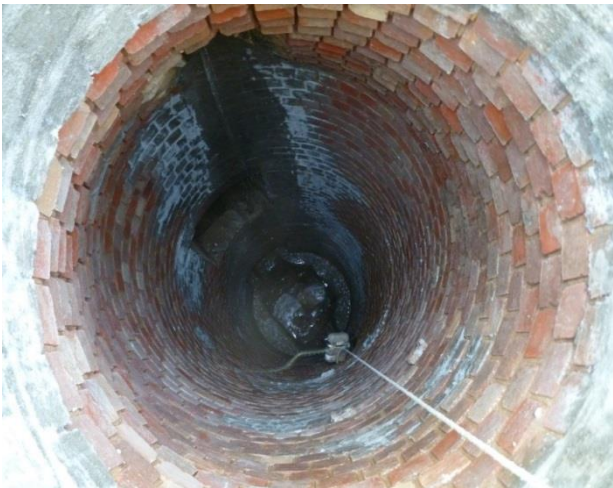
Figure 16: Brick manhole with lime mortar degraded from H 2 S attack
