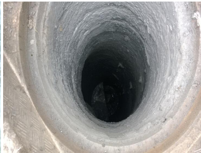
Figure 16: Brick manhole with lime mortar degraded from H 2 S attack
