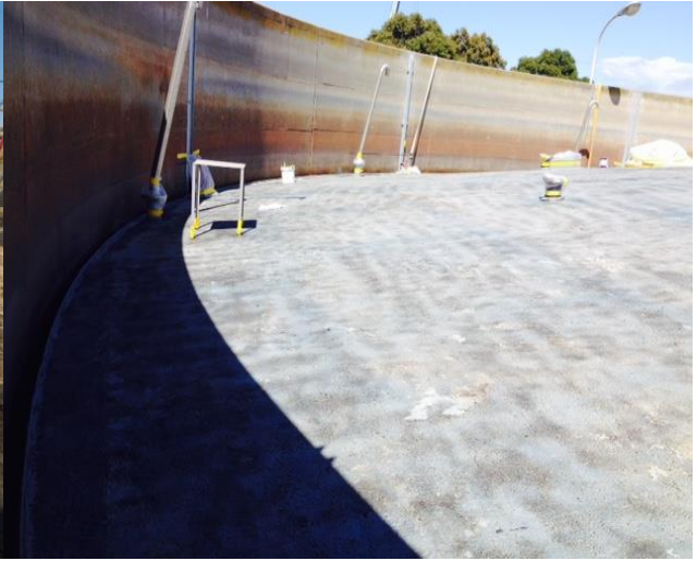
Figure 9: Prepared substrate with primer applied
