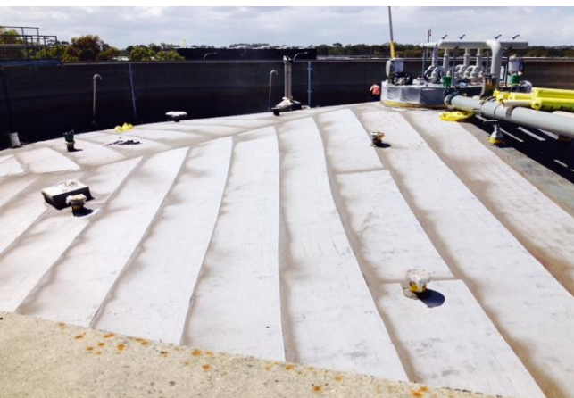
Figure 12: Geotextile installed, awaiting top coat
