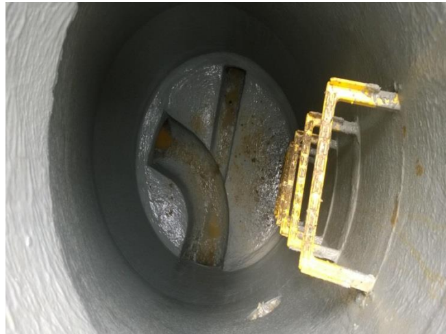
Figure 17: Manhole relined with Advanced Cementitious Coating
