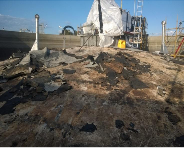
Figure 8: Old membrane being removed
