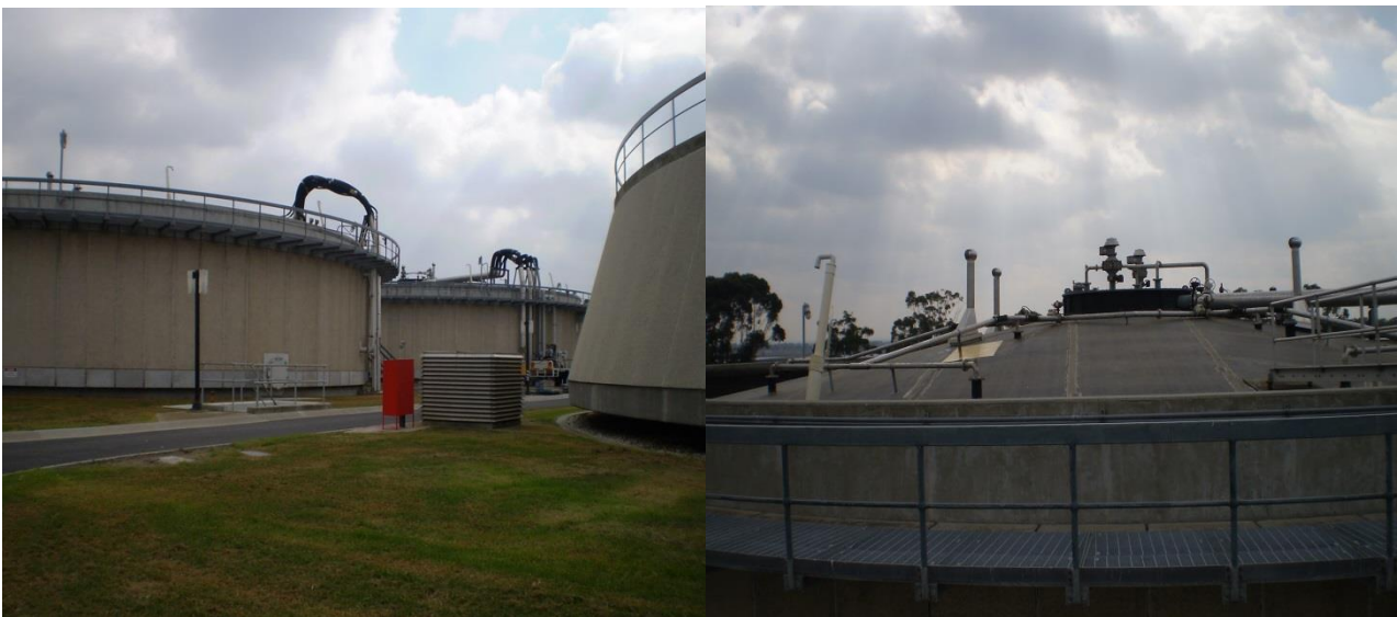
Figures 6 & 7: Overview of the digester
