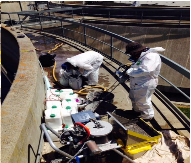
Figure 11: Mixing the waterproofing membrane
