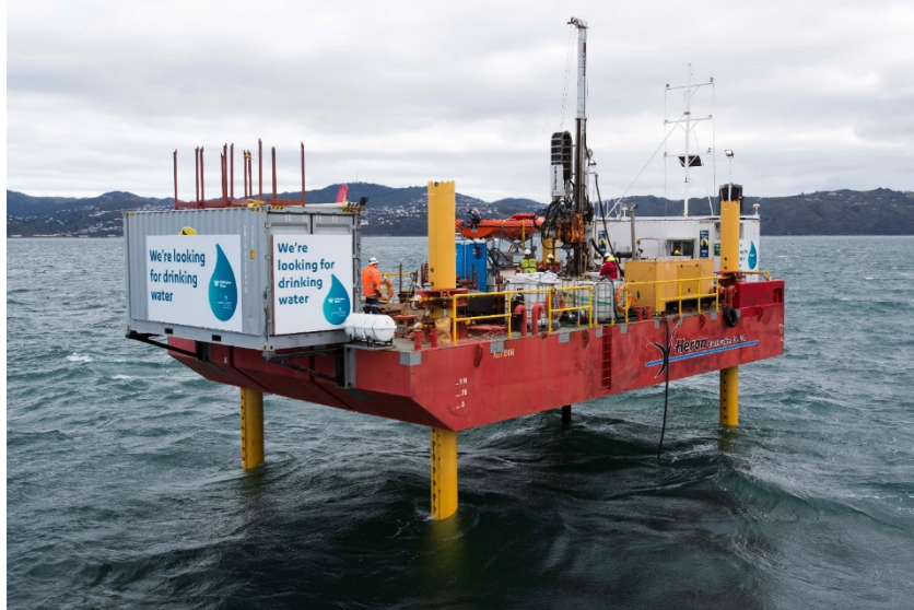
Figure 3 Jack-up barge in action
