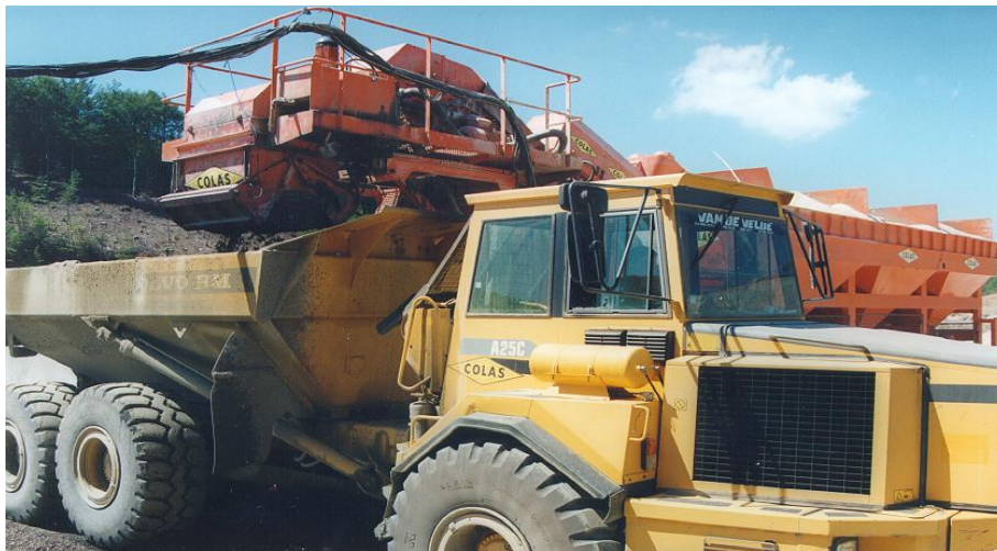
Figure 5: Cold asphalt plant on site
