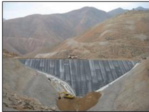
Figure 14b: Upstream face after BGM installation
