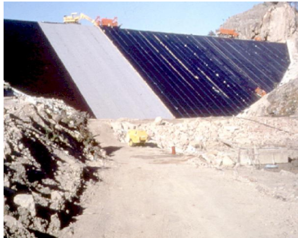
Figure 11b: Ortolo dam
