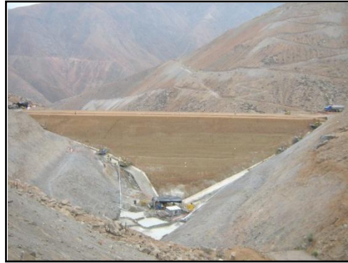
Figure 14b: Upstream face after BGM installation
