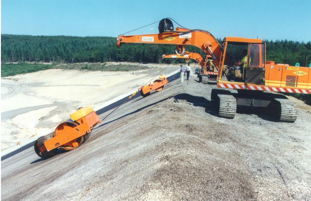
Figure 2: Compaction of the rockfill
