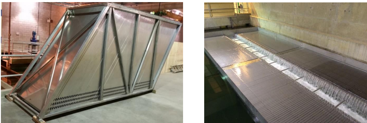
Figure 4: Parallel plate settler pack retrofit
