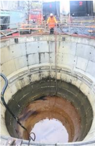
Figure 16: ground water in caisson
