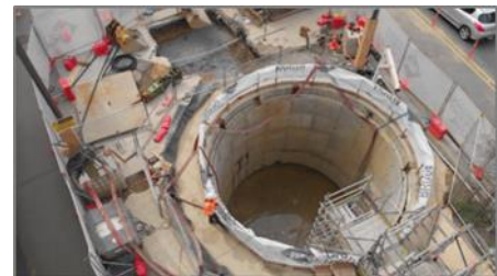
Figure 21: Caisson from above
