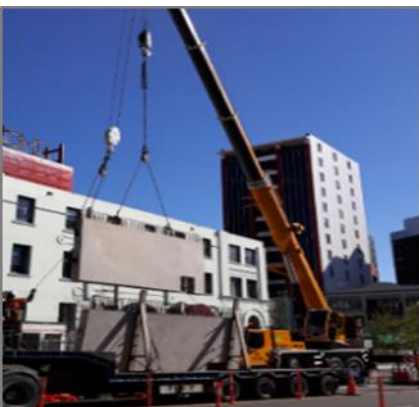
Figure 19: Mobile crane placing wall panel
