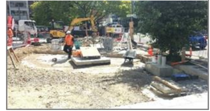
Figure 24: WCC trees adjacent to pump station
