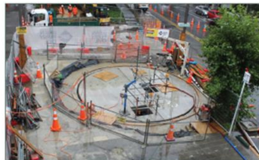
The pump station chamber, now covered.
