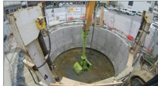
Work on the pump station chamber
