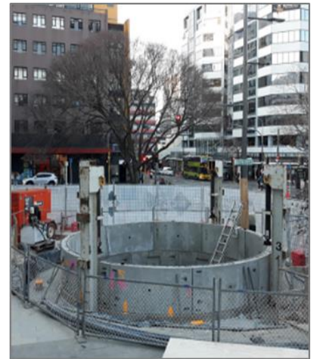
Figure 17: 4 No. 25tonne hydraulic jacks
