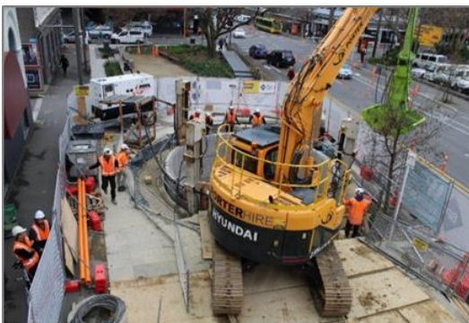
Figure 8: Construction within restricted site compound
