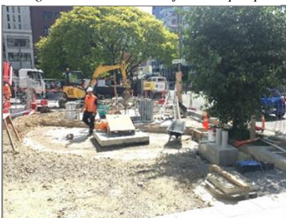
Figure 22: WCC trees adjacent to pump
