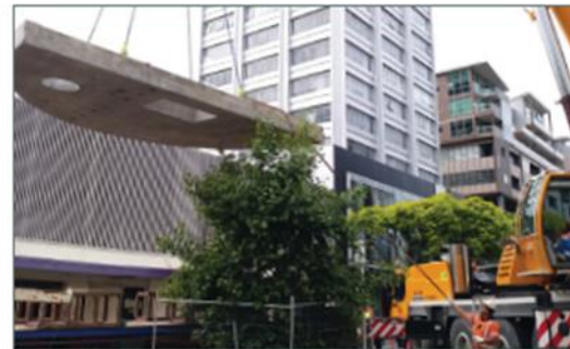
Craning the second of two large roof slabs into place.
