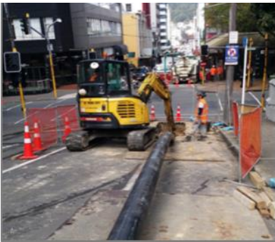
Figure 20: 3tonne excavator working in Willis Street
