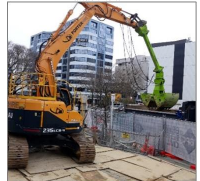
Figure 18: 24tonne excavator with clamshell attachment
