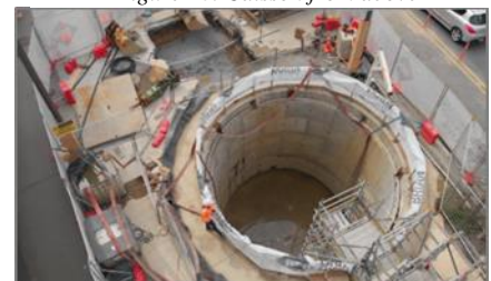
Figure 26: Caisson from above
