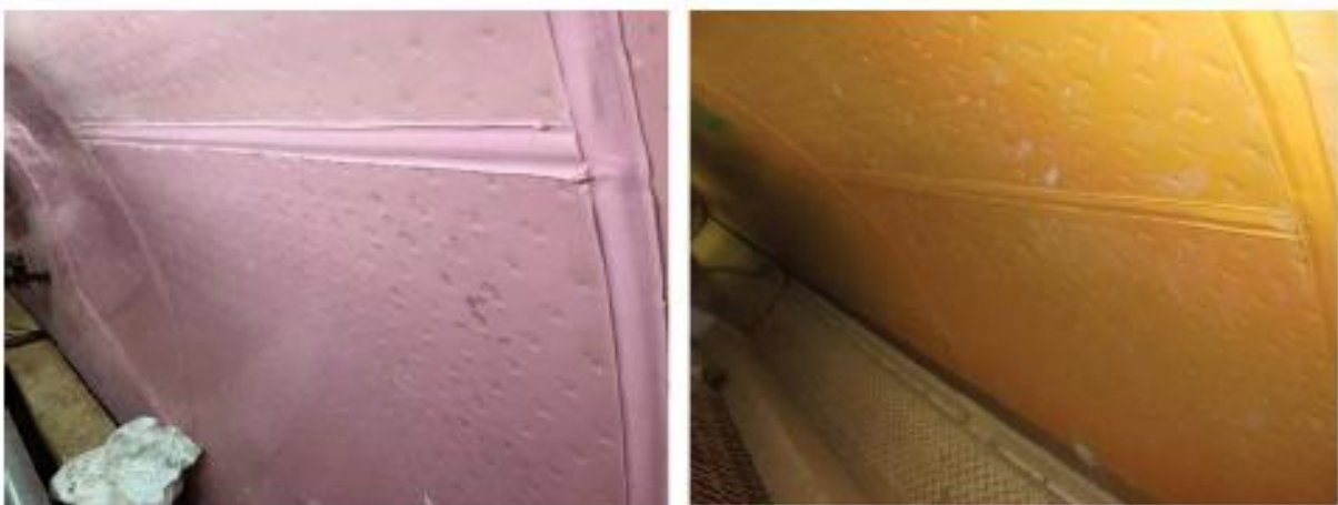
Photograph 4: Radial Joint Welds on Plastic-Lined Segmental Linings from Doha
