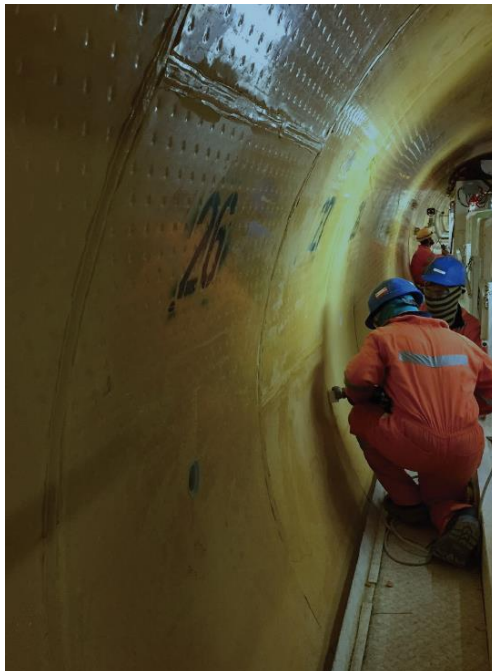
Photograph 4: Radial Joint Welds on Plastic-Lined Segmental Linings from Doha
