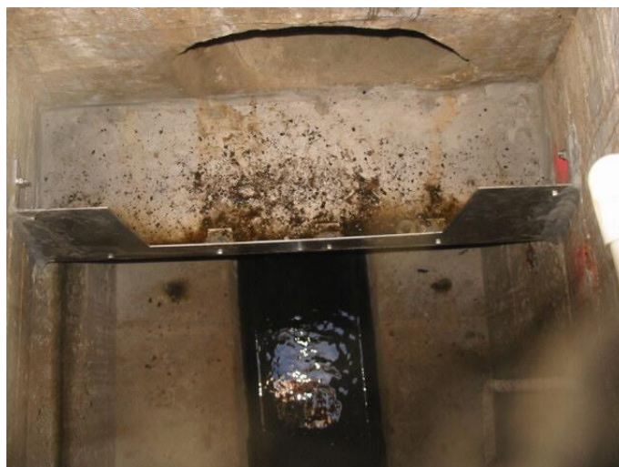
Photo 1: Sewer manhole with overflow weir installed
