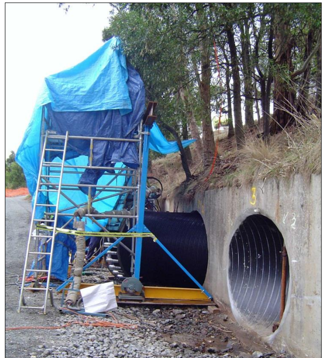
Figure 9: Installing a Ribline liner in an 1830mm diameter culvert. Note the culvert in the foreground has been completed, including grouting and epoxy end sealing.
