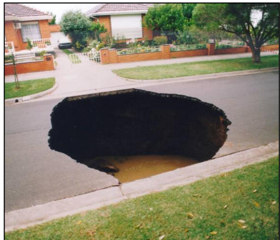
Figures 3 and 4: Road collapses caused by embedment being washed into a deteriorated or defective culvert or pipeline, leading to the formation of voids beneath the surface.
