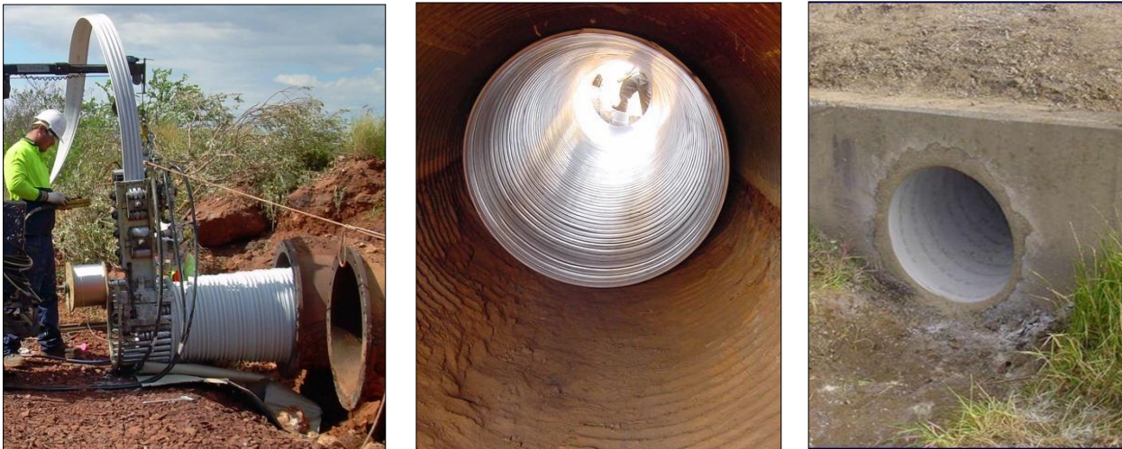
Figure 6: Installing Expanda Pipe in under-road and rail culverts
