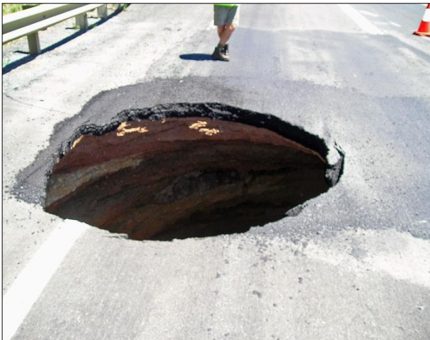
Figures 3 and 4: Road collapses caused by embedment being washed into a deteriorated or defective culvert or pipeline, leading to the formation of voids beneath the surface.
