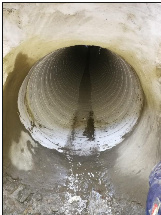
Figure 11: Expanda Pipe liner installed restores structural capacity. Curved invert reduces siltation
