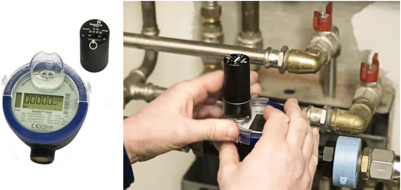
Figure 11 Mounting of the “Optical Eye”
