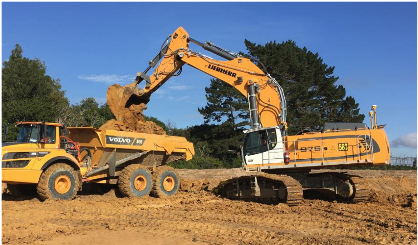
Figure 4.1: Wetland excavation using 3D machine control systems
