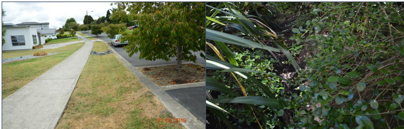
Photographs 9 & 10: Swale 2 Residential Subdivision & Swale 3 single lot bush swale
