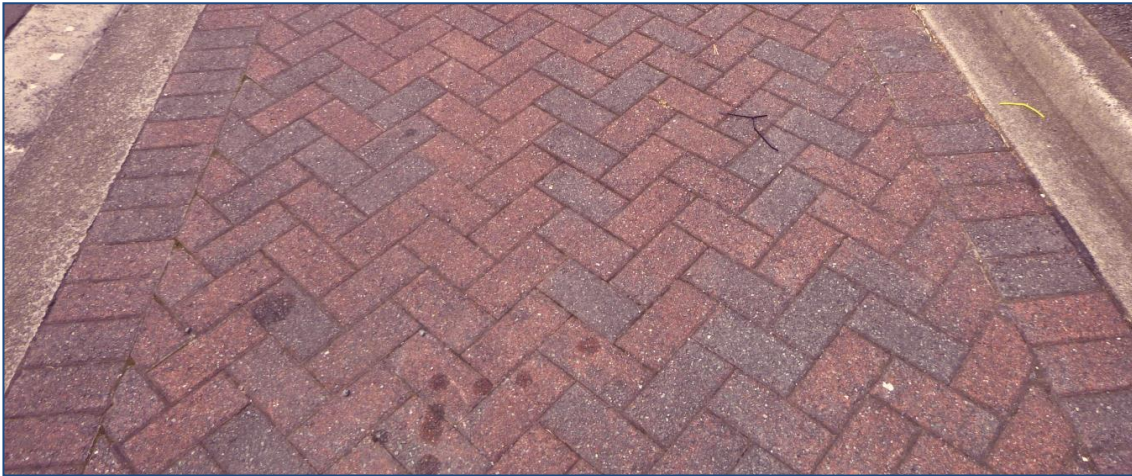
Photographs 18: Permeable Paving 3
