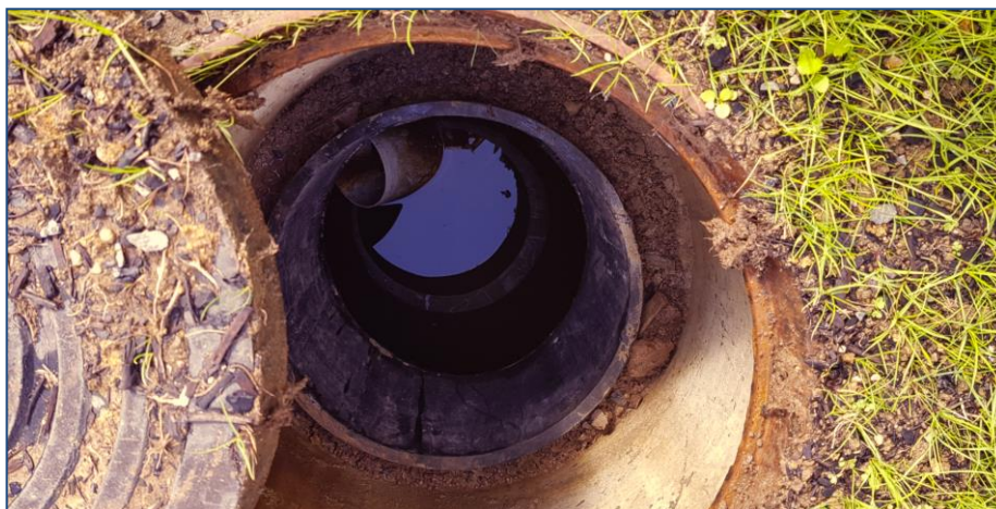
Photographs 19: Underground Tank 6
