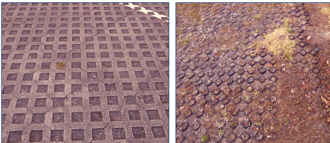
Photographs 16 & 17: Permeable Paving 2
