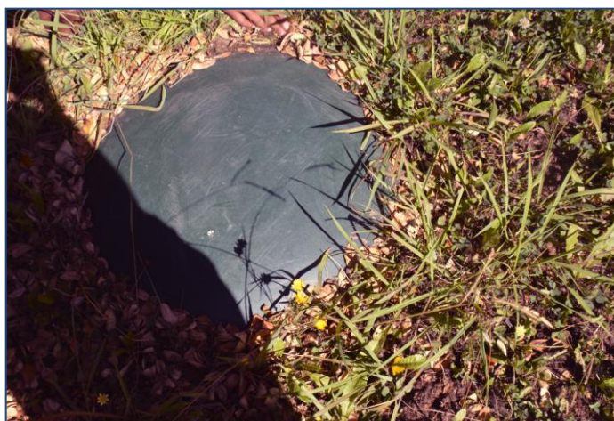
Photographs 20: Typical Underground Tank 7-19
