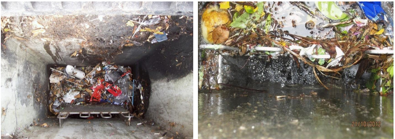
Figure 2 TetraTrap pollutant capture (dry and wet conditions)
