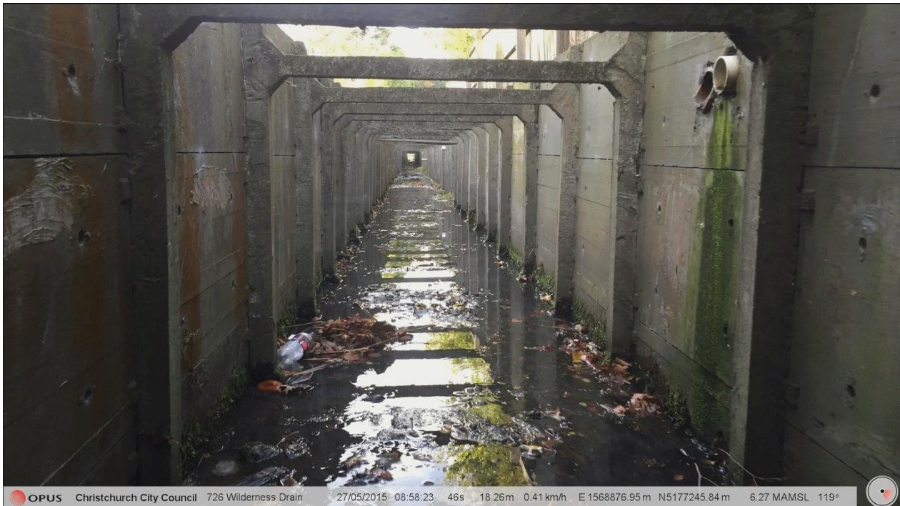
Figure 3: Geo-referenced video screenshot. The field on the bottom identifies data in the video such as distance from the upstream point, speed, GPS location, elevation (estimate), and direction.
