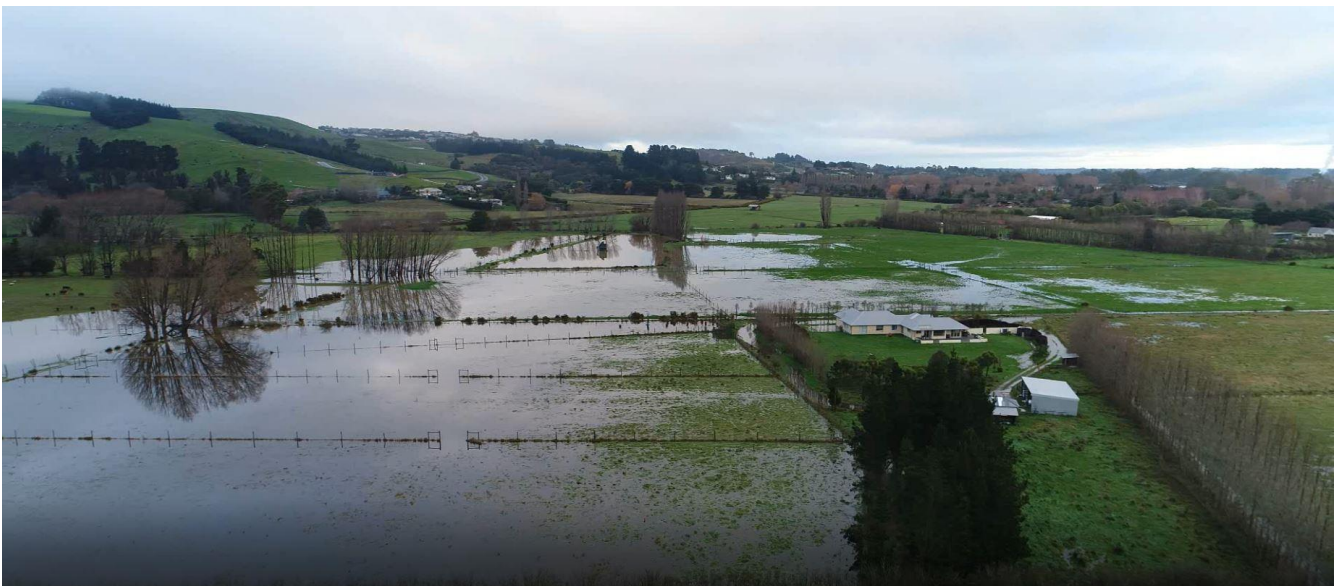
Figure 4: A snapshot of the aerial footage taken on the 23 rd of July 2017 looking from the constructed Eastman Wetlands toward the proposed Sutherlands Basins.
