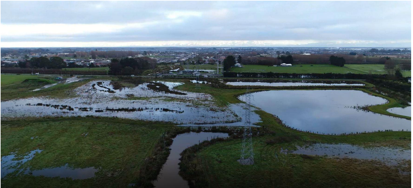
Figure 3: A snapshot of the aerial footage taken on the 23 rd of July 2017 looking at the constructed Eastman Wetlands.
