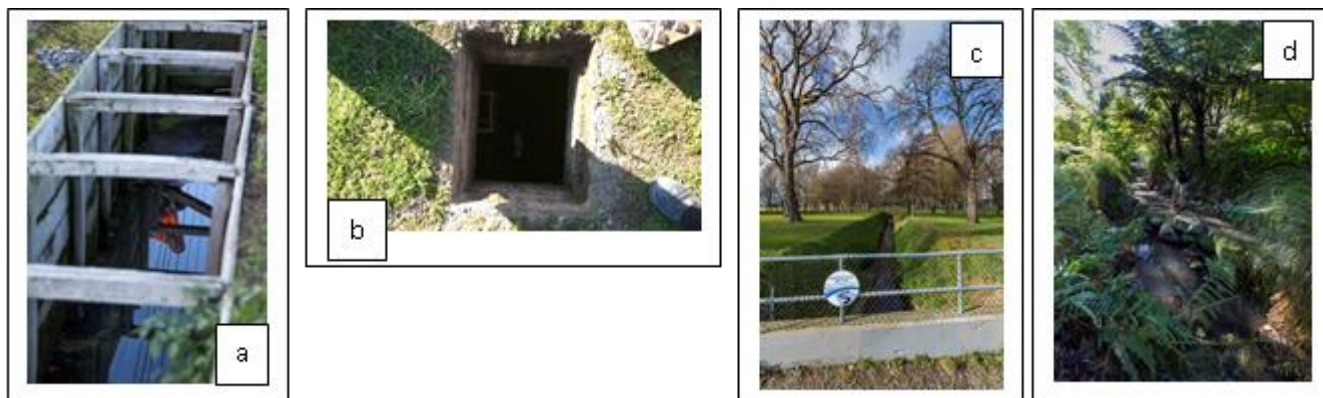
Figure 2. Photos of Addington Brook throughout the catchment (a) timber-lined box drain upstream of Matipo Street stormwater ponds (b) view down stormwater sump to the piped brook in mid-catchment (c) stream as reemerges through Hagley Park (d) section of stream through the Botanical Gardens
