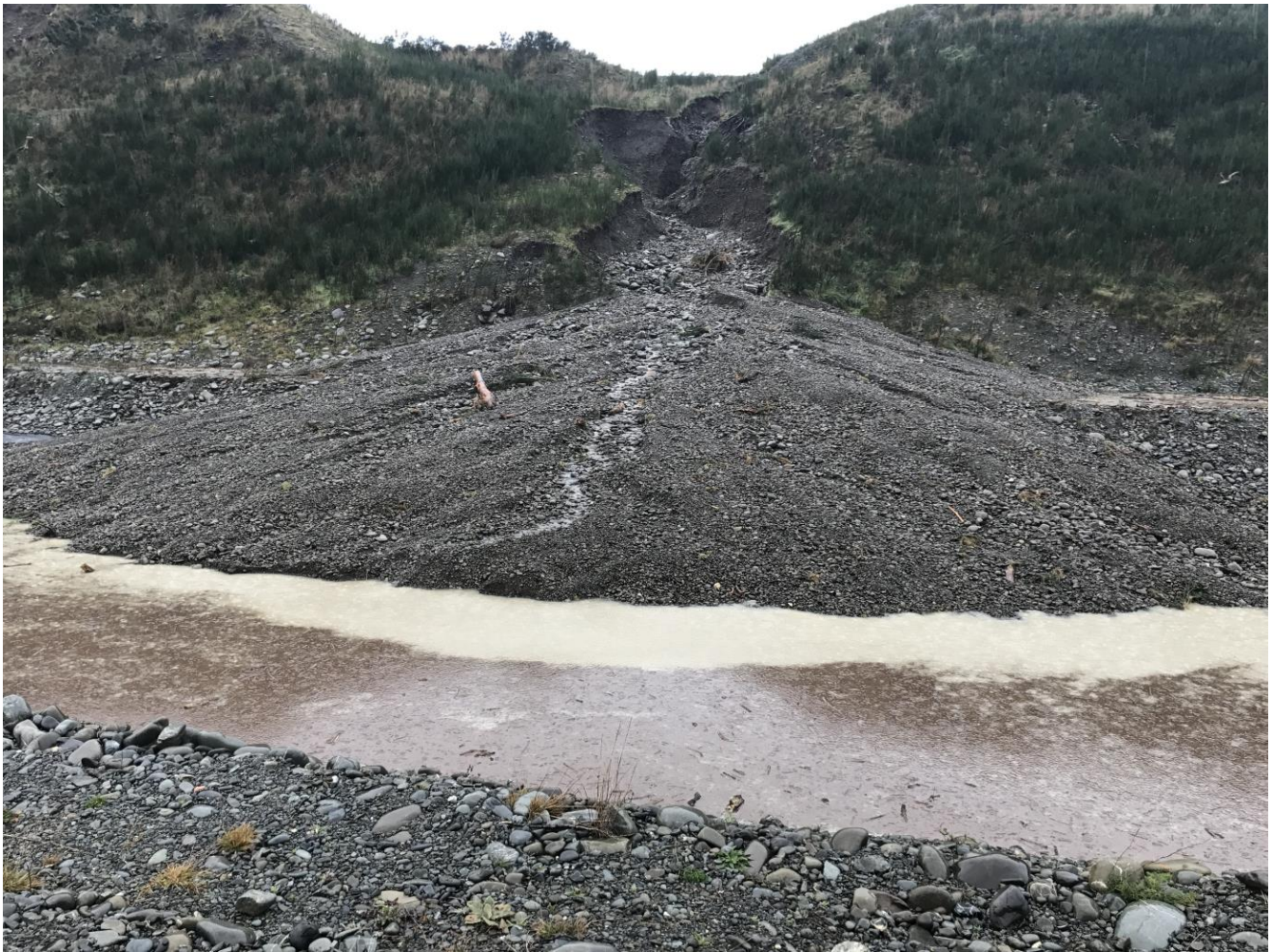
Photograph 1: The slip prior to remediation
