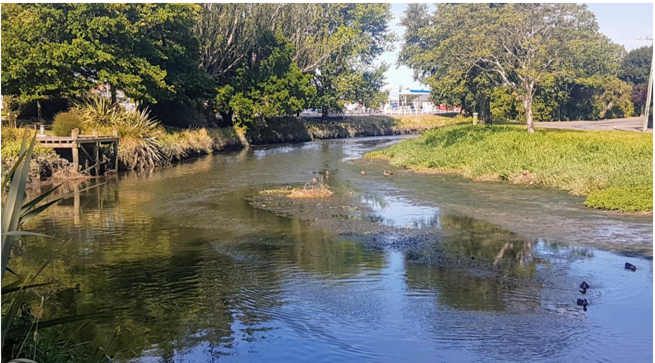
Photograph 2: Siltation of the Ōpāwaho / Heathcote River showing reduced channel capacity
