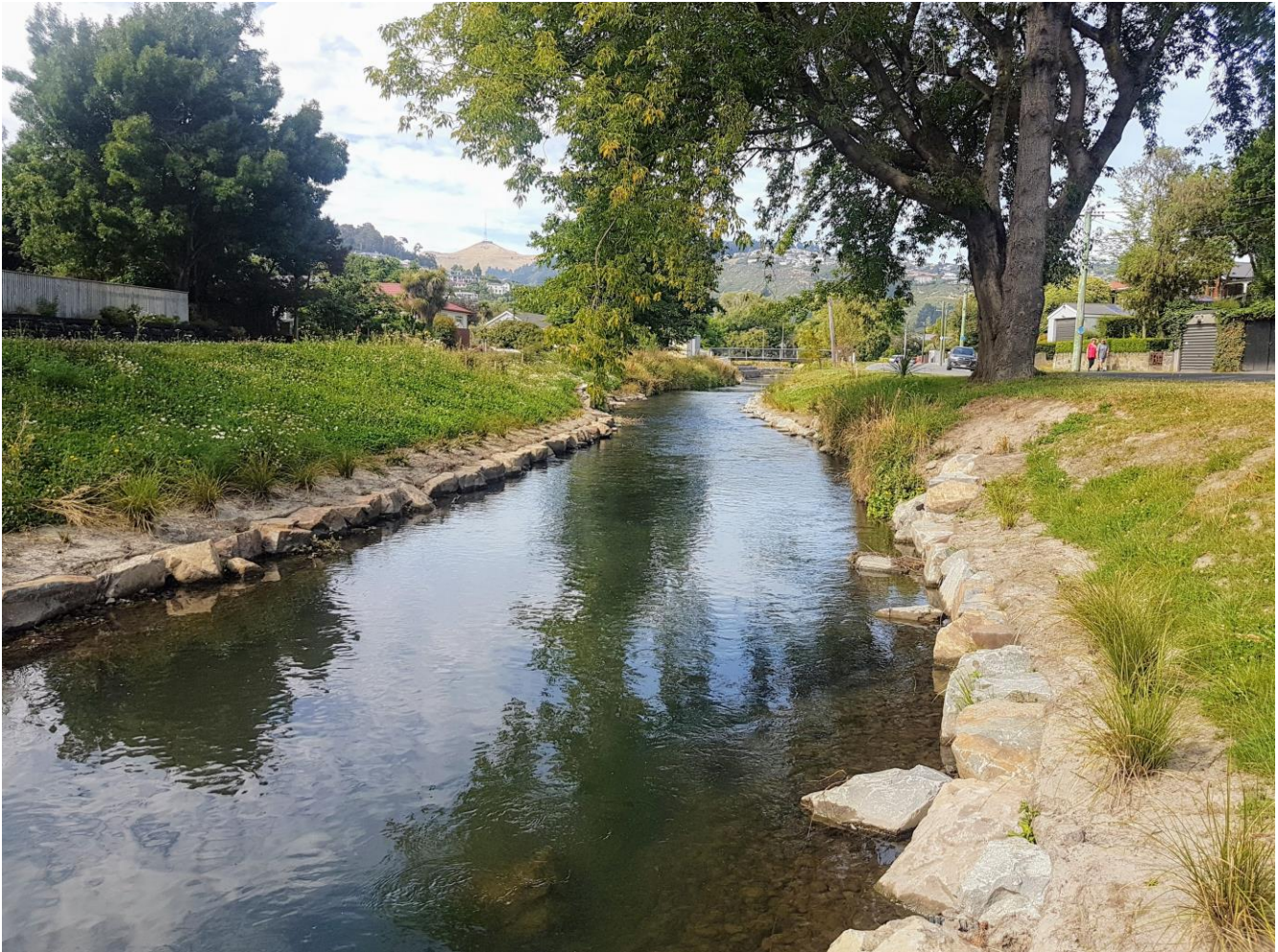
Photograph 3: Completed bank stabilisation showing increased channel capacity
