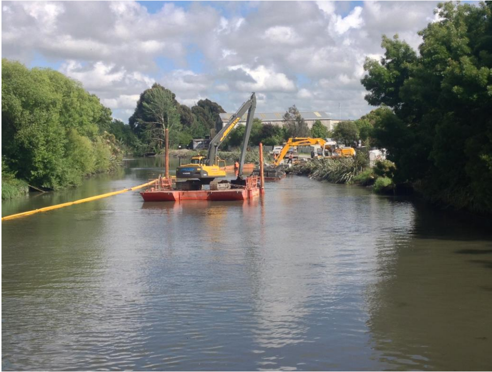
Photograph 4: Dredging by barge operation (Stage 1)
