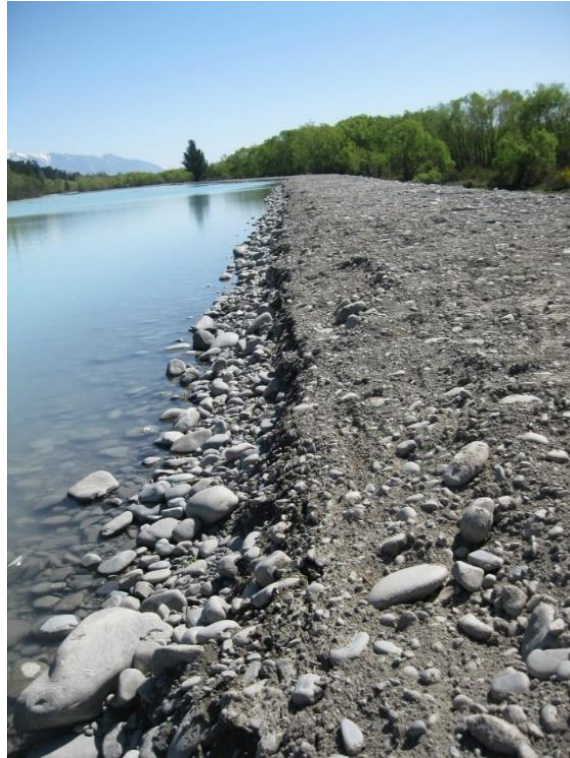
Photograph 3: Beach formed in sandy gravel protection layer (example – not from Heathcote River)
