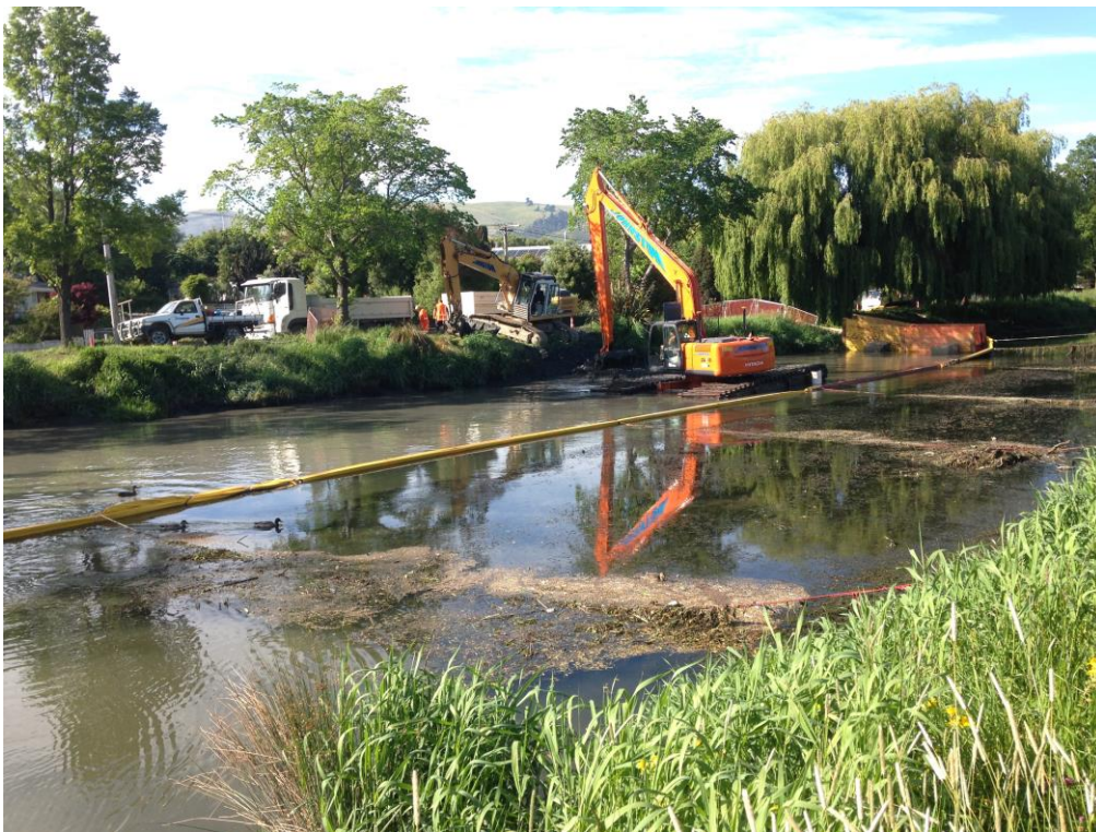
Photograph 5: Dredging by long reach and amphibious excavators (Stage 2)
