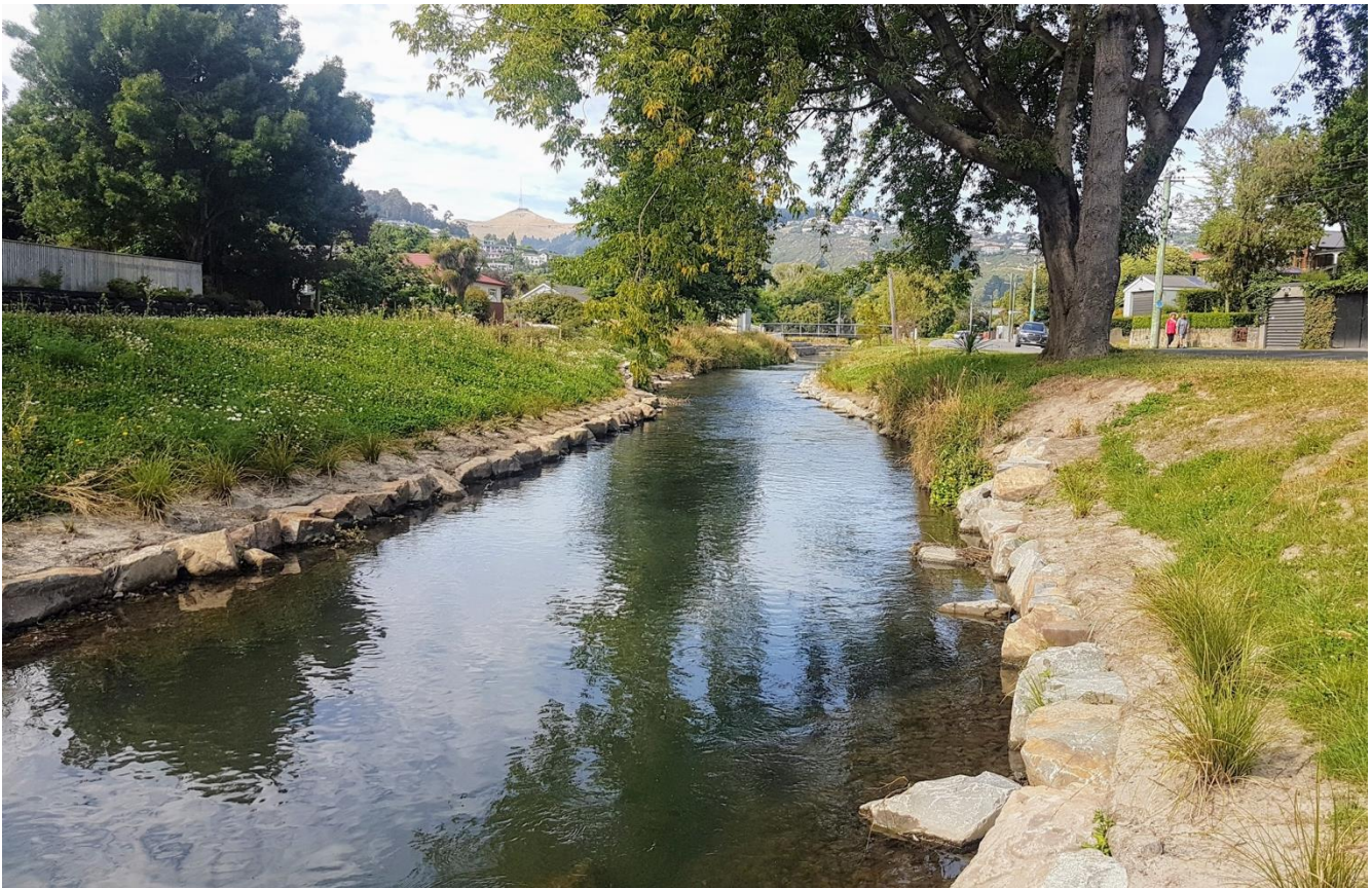
Photograph 4: Completed bank stabilisation showing increased channel capacity
