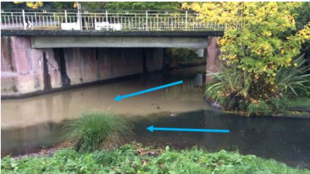
Photograph 2: Confluence of Cashmere Stream (high sediment load) with an urban stream in May 2017 (image source unknown)
