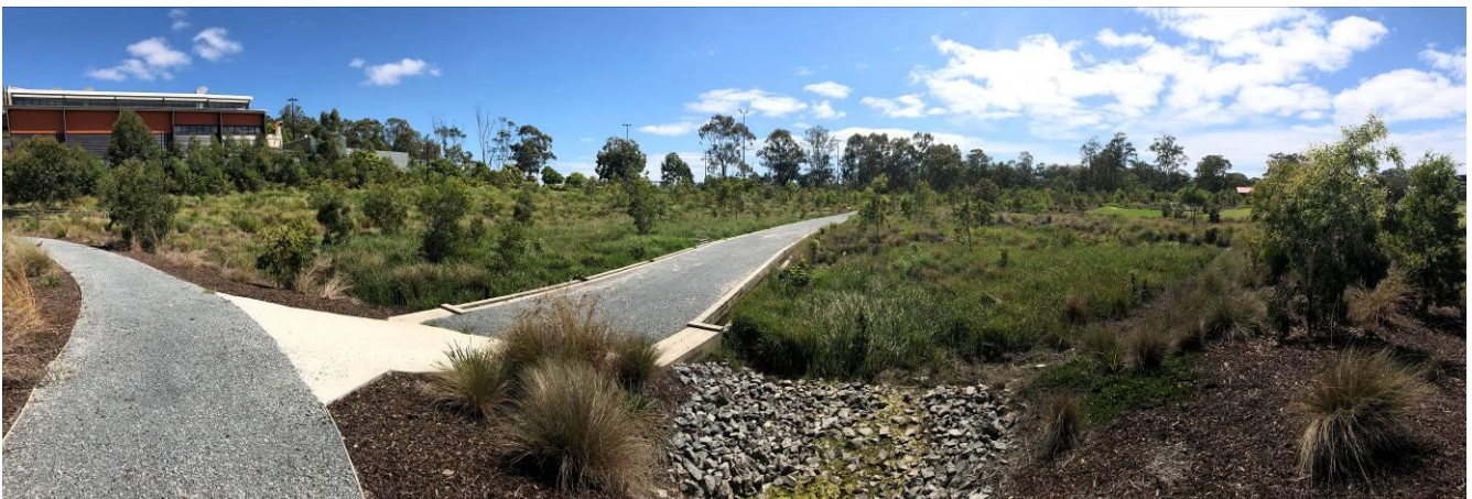
Figure 4: Large biofilter at the Gold Coast commonwealth games village where extended detention is shared with an inlet pond and biofilter surface
