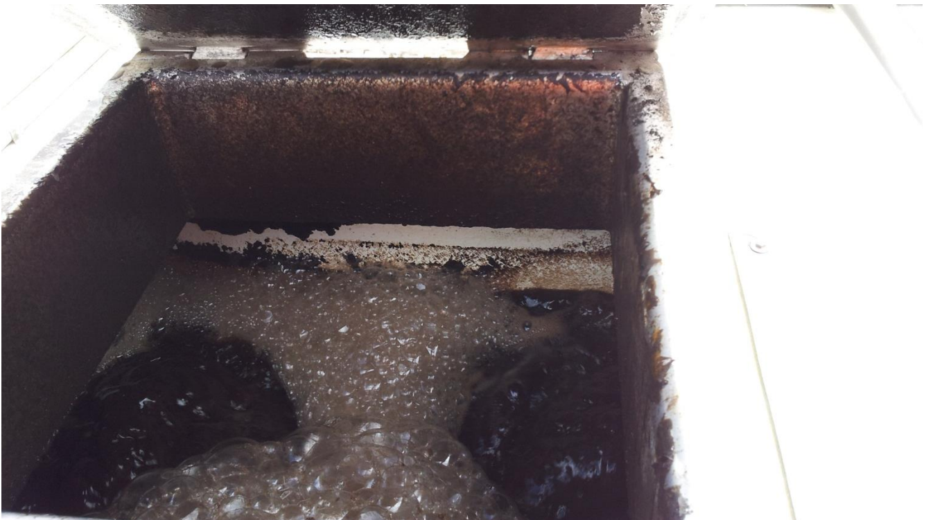
Photograph 6: Full scale treatment plant SAF tank foaming
