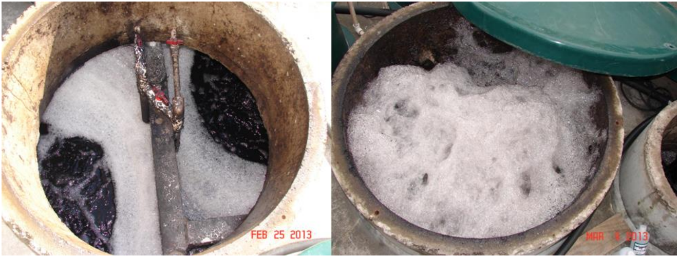
Photographs 1 & 2: Foam production observed during the trial in the main chamber of the SAF unit
