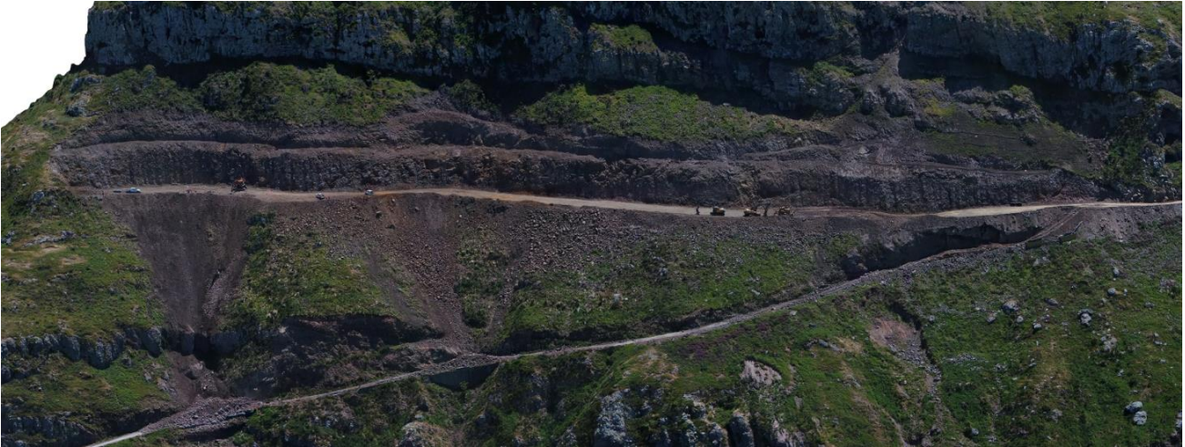
Figure 3: Catch Bench Construction
