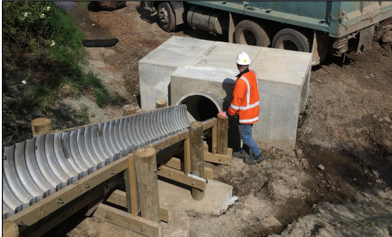
Figure 16: Gullies Energy Dissipation Structure
