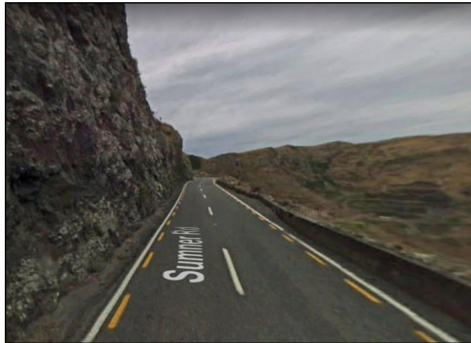
Figure 5: Typical view of the upper part of the road with cliff and hand formed channel on the left and rockwall on right (sea side). (Source: Google Streetview).
