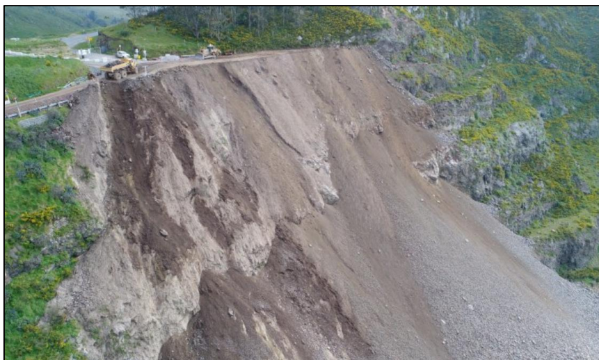
Figure 8: Gollans Bay/Evans Pass Tiphead Prior to Rehabilitation (Source: Doug Hood Mining)
