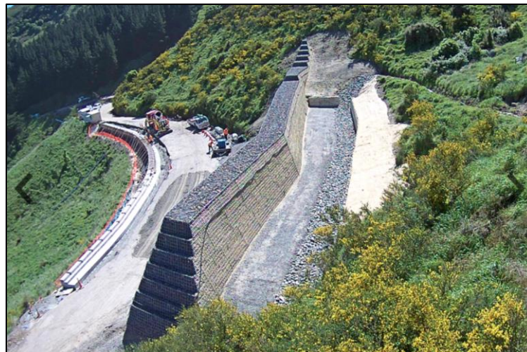
Figure 4: Rockfall Interception Bund in F Gully Prior to Revegetation (Source: MCD)
