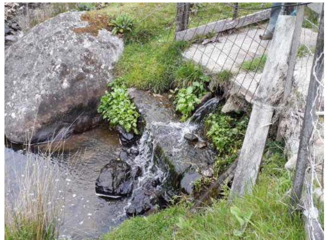
Figure 4-4 Existing low flow outlet
