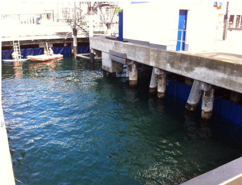
Photograph 5: The completed baffle
