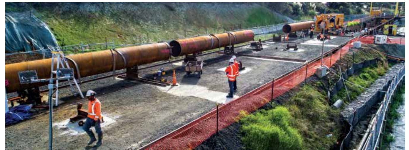
Below: The Herrenknecht Direct Pipe TBM being assembled.
