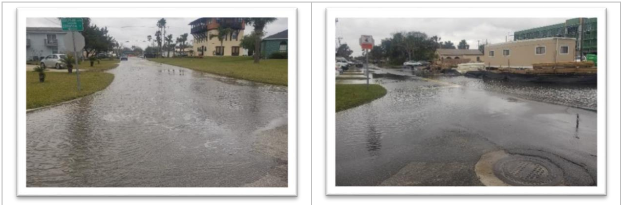
Flooding occurring due to an unprotected outfall not owned by the City.
