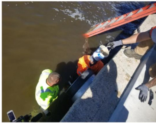
Installation of a WaStop check valve DN750 (30").
