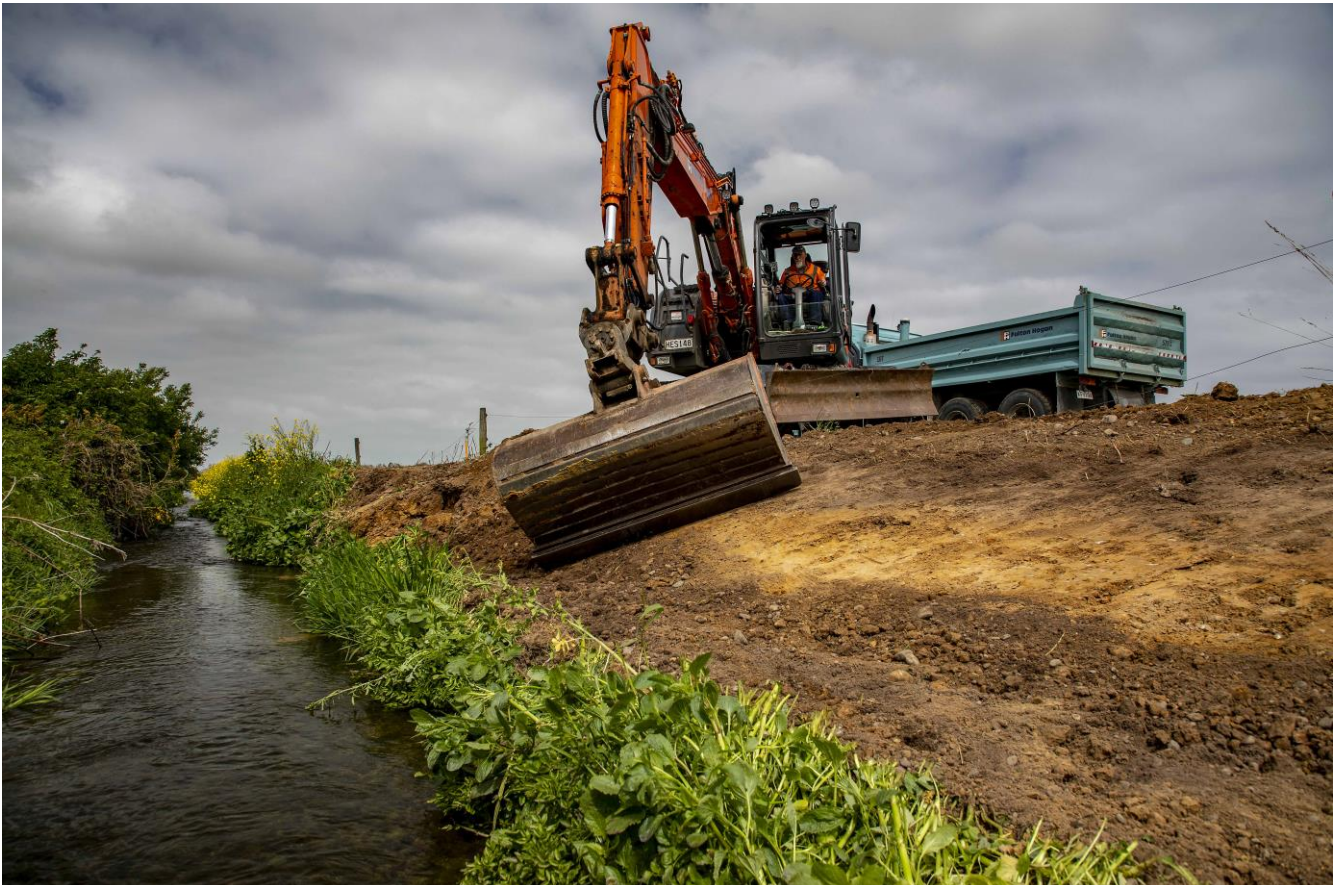
Photograph 3: Reshaping the over-steepened banks
