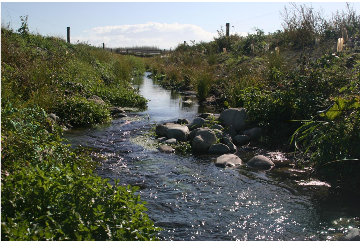
Photograph 4: View of Snake Creek Rock Features and Planting
