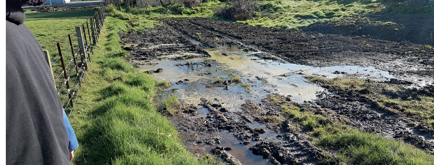
Failed onsite wastewater system land application. A serious health risk.
