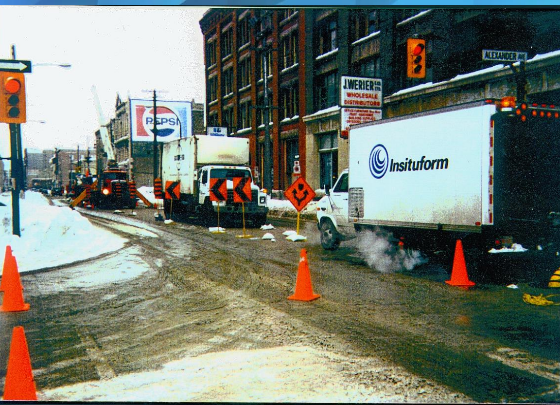
General Site Setup and Inversions of 600 mm (24") Installation on Princess - 1994
