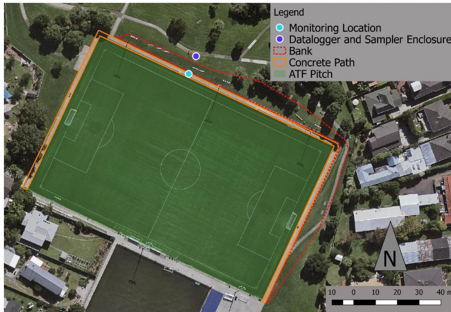
Figure 2. Contributing catchments for the Michaels Ave ATF (aerial photo from Auckland Council)
