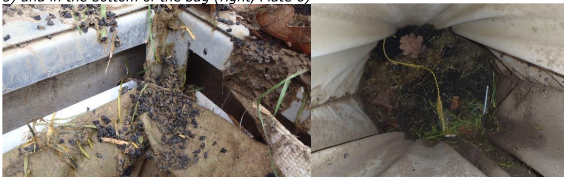
Plates 3-6. Above, a catchpit grate on the concrete path (left, Plate 3) and the Enviropod filter bag (right, Plate 4). Below, crumb rubber deposited within the Enviropod filter bag overflow (left, Plate 5) and in the bottom of the bag (right, Plate 6)
