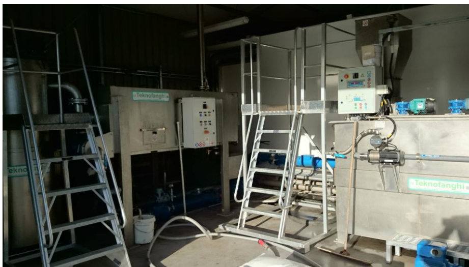
Photograph 1: Recuperative Thickener Installation (Photograph was taken during construction)
