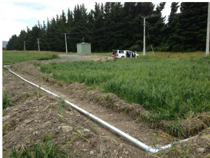
Photograph 12: Existing rising main from bores temporarily redirected around construction site
