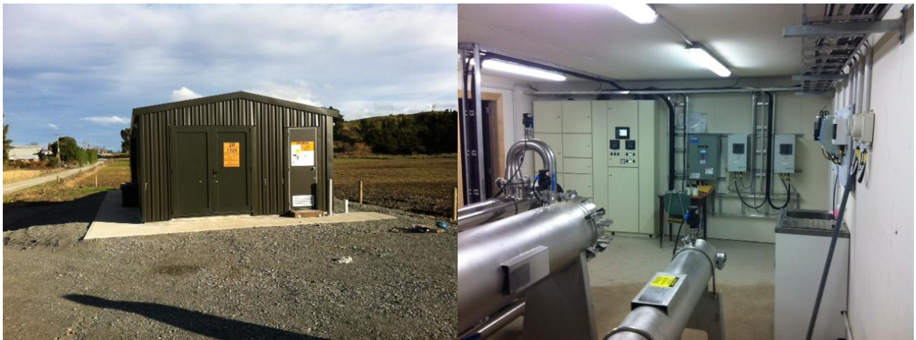
Photograph 6: Mossburn Treatment Plant (Upgraded)
