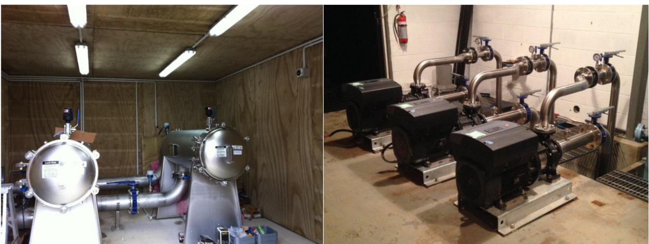
Photograph 8: Winton Treatment Plant (Upgraded)
