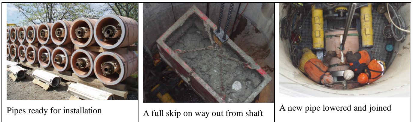
Figure 5: Microtunnelling construction photos
