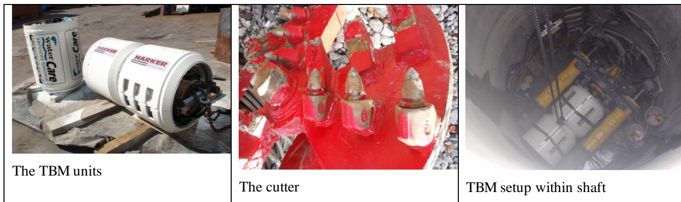
Figure 4: Microtunnelling equipment
