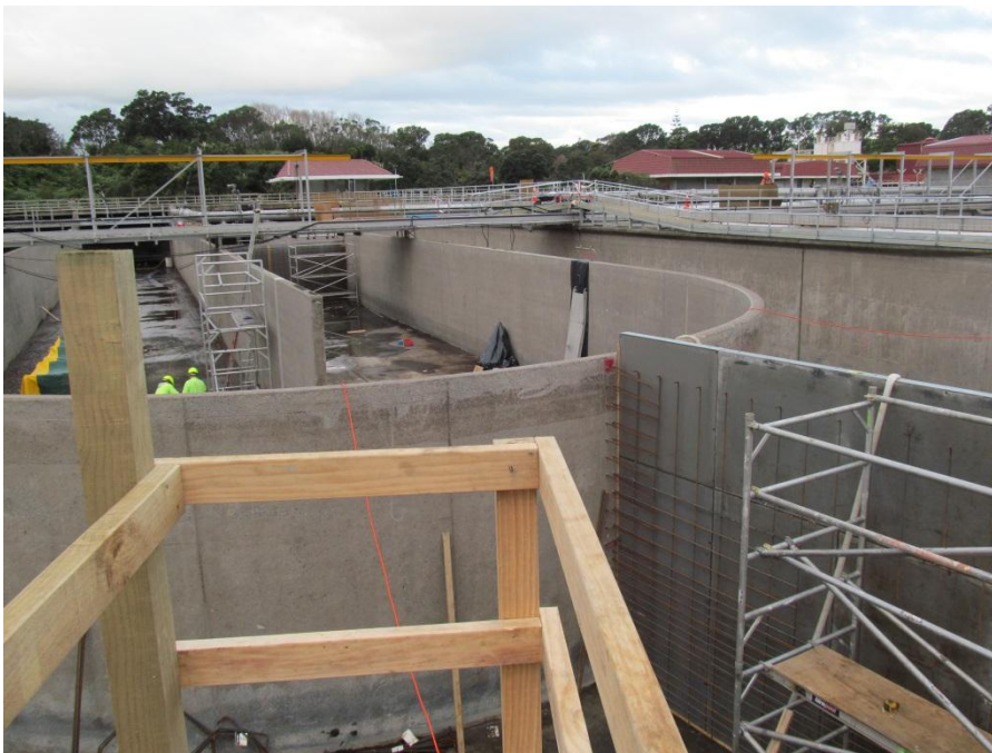
Photograph 1: Construction of the partition wall in Bioreactor 2
