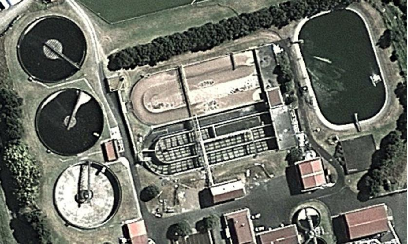
Photograph 3: Google Earth view of the New Plymouth WWTP during installation of diffuser grids on Bioreactor 1.
