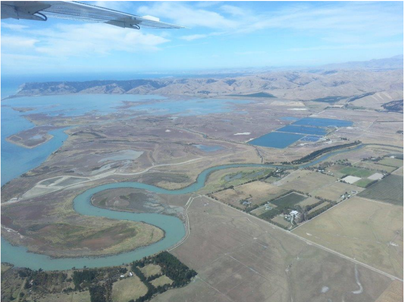
Figure 8: View looking south with construction underway of the long wetlands with Opawa River in foreground and Wairau Lagoons upper left and the STP ponds upper right.
