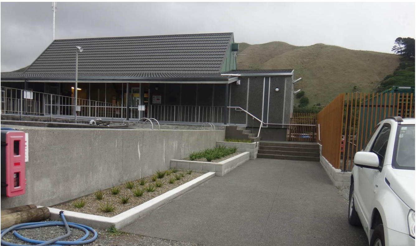
Photograph 10: Upgraded Operations Building
