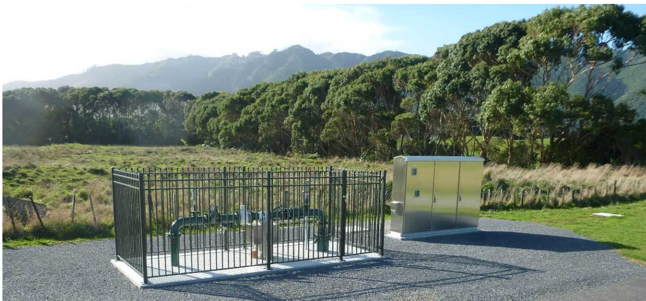
Photograph 12: New Bore Kb7 Installation
