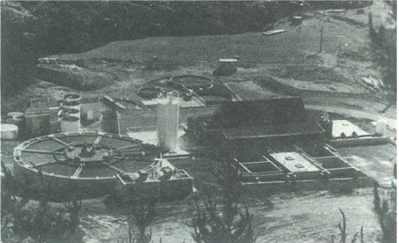
Photograph 1: Waikanae Water Treatment Plant. Completed March 1977 (Source New Zealand Engineering Vol 33 No. 1 1978)
