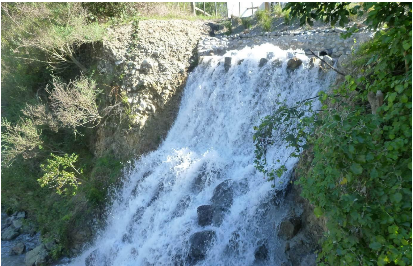
Photograph 15: New River Discharge Structure
