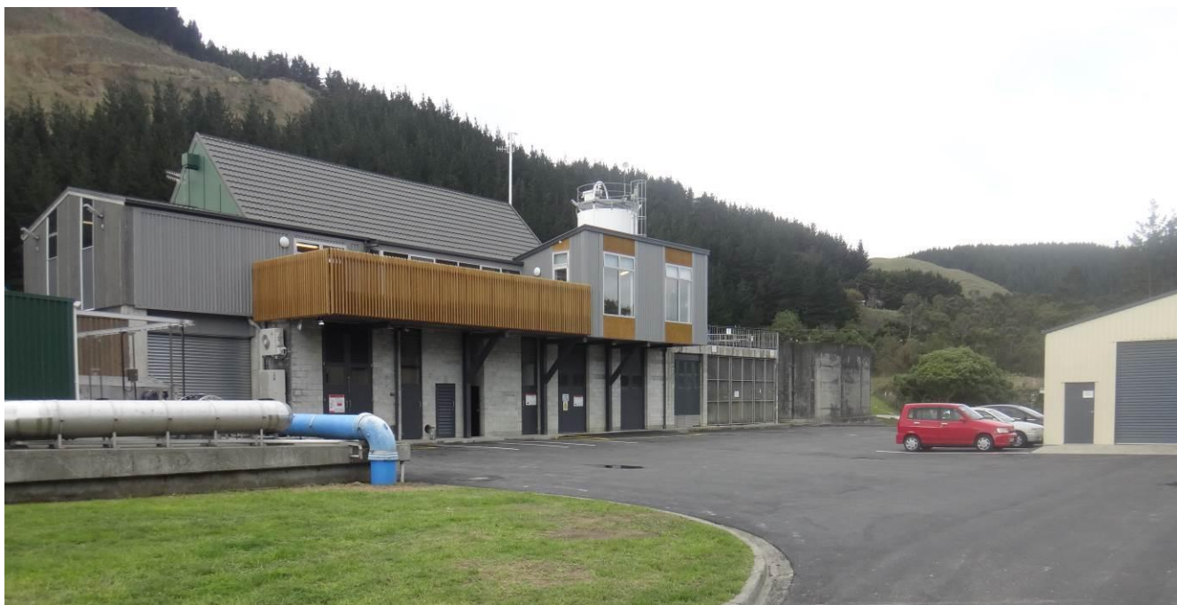
Photograph3: Upgraded Operations Building, Completed May 2015
