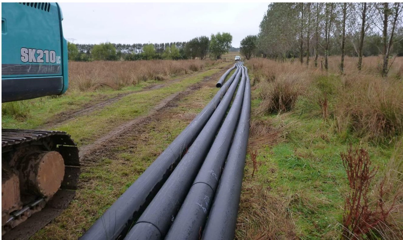
Photograph 13 Pipe Strings Prepared for Installation
