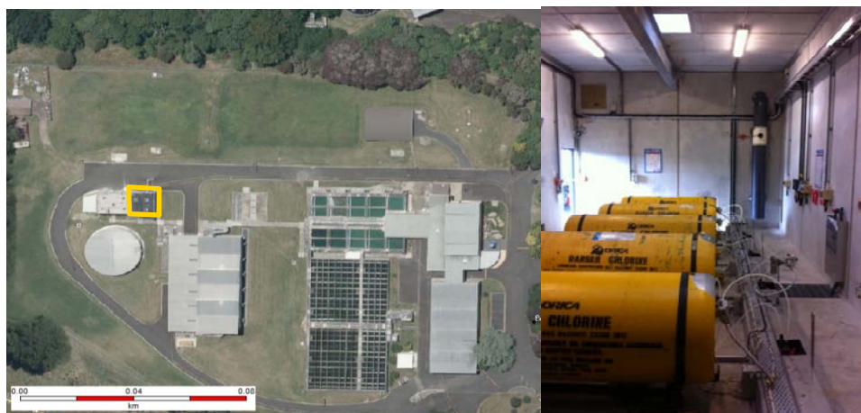
Figure 2: Existing WTS Layout and Chlorine Drum Store Room
