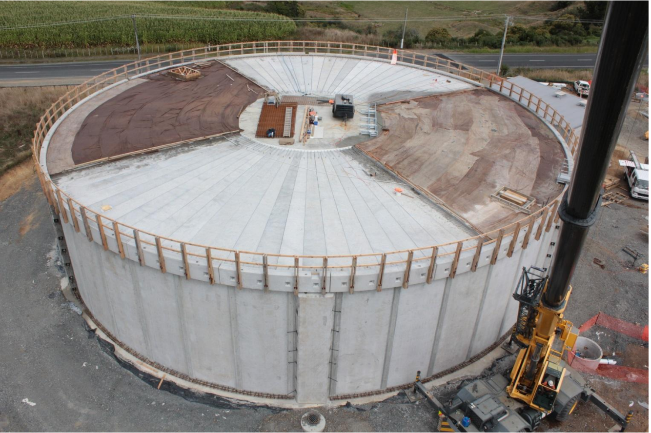
Figure 2: Reservoir Nearing Completion
