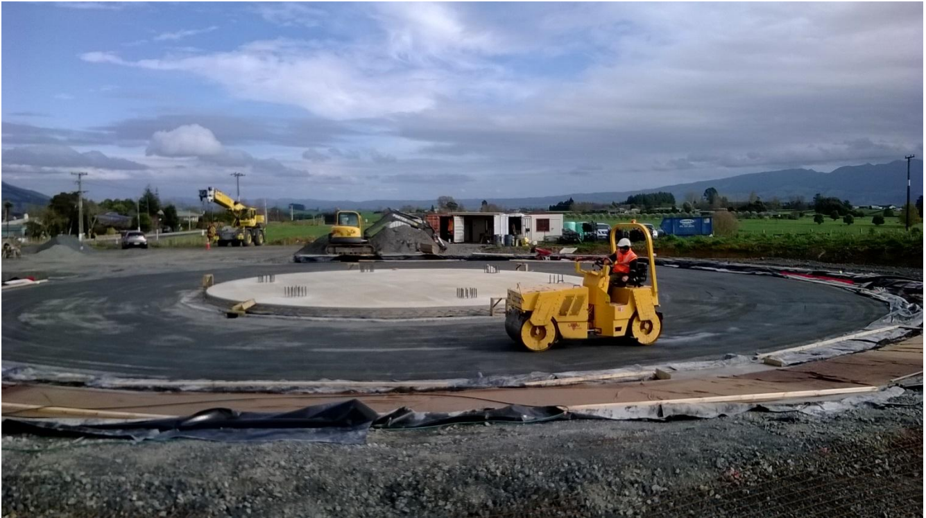
Figure 1: Reservoir Foundation Being Prepared Following Preload
