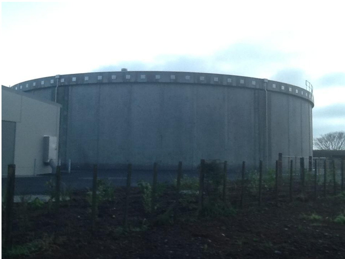
Figure 3: Reservoir complete and in operation
