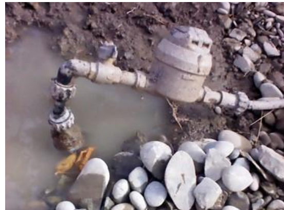
Figure 10. Damaged compression fitting assembly (Citycare)
