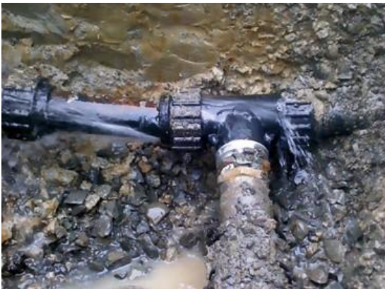
Figure 9. Leaking compression fitting assembly (Citycare)
