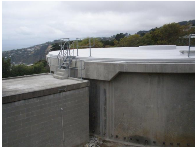
Photograph 6: Upper Balmoral Reservoir Ring Beam and Roof Membrane
