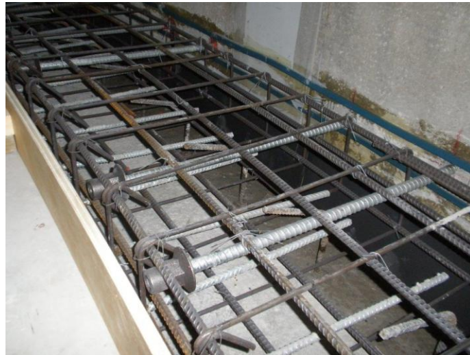
Photograph 8: Shear Connection Wall to Floor Slab
