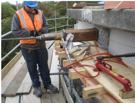
Photograph 4: Upper Balmoral Reservoir Testing Anchorages for Ring Beam
