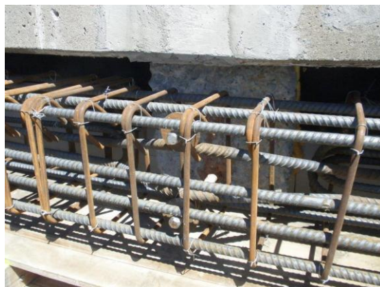
Photograph 5: Upper Balmoral Reservoir Ring Beam Reinforcing
