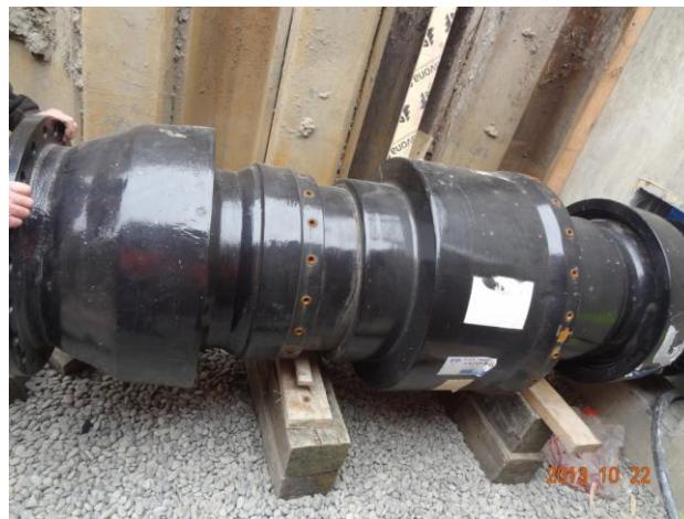
Photograph 10: EBAA Flex-tend Fitting (PS105)
