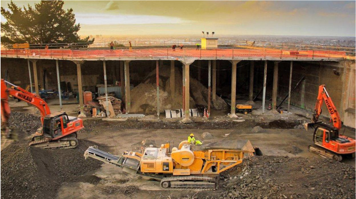
Photograph 2: Huntsbury No. 1 Stage 2 Reservoir – Under Construction
