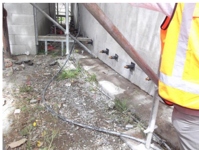
Photograph 7: McCormack's Bay Shear Connection Wall to Floor
