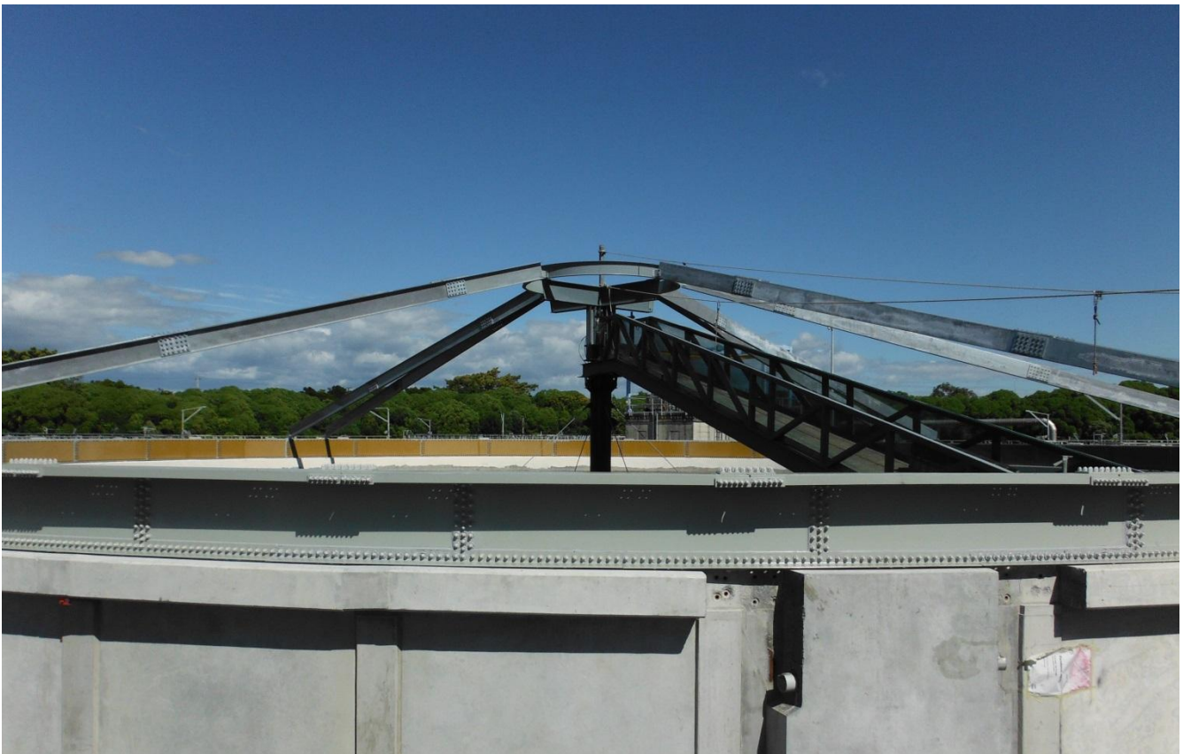
Figure 8 - Gantry Structure Used to Assist Roof Installation
