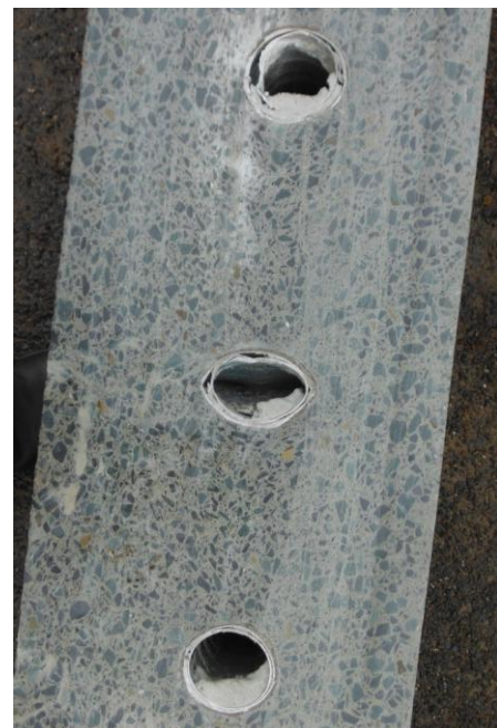
Figures 4A and 4B - Saw Cut Removed Stitch Showing Duct Deformities
