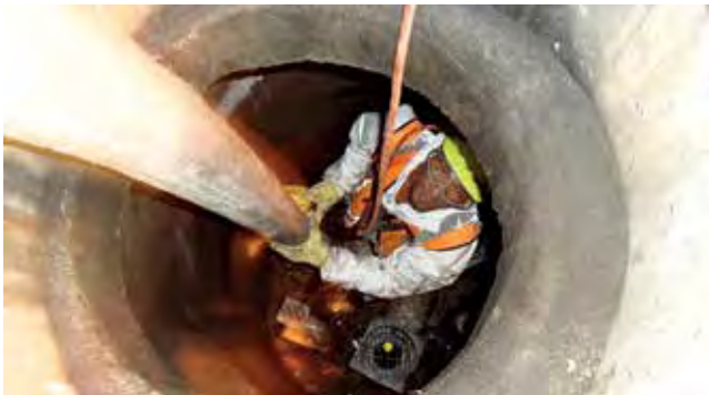
SH1 Khyber to Gillies Soakage Inspection, Peter Mitchell.
