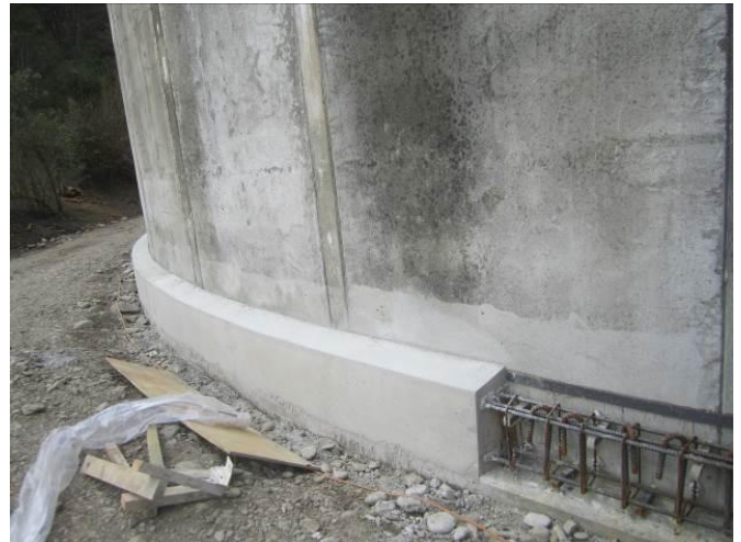
Photographs 4 and 5: Inserted dowels at Champion Road (left) and beam construction at Queen Street (right)
