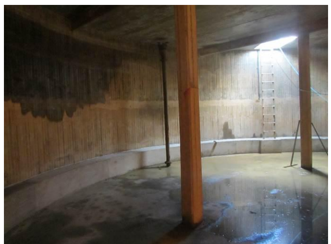
Photographs 6 and 7: Internal strengthening works at Valhalla Lane reservoir
