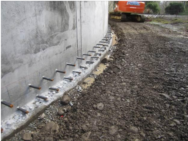
Photographs 4 and 5: Inserted dowels at Champion Road (left) and beam construction at Queen Street (right)
