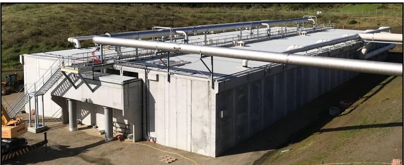
Photograph 6: Contact Stabilisation Tanks
