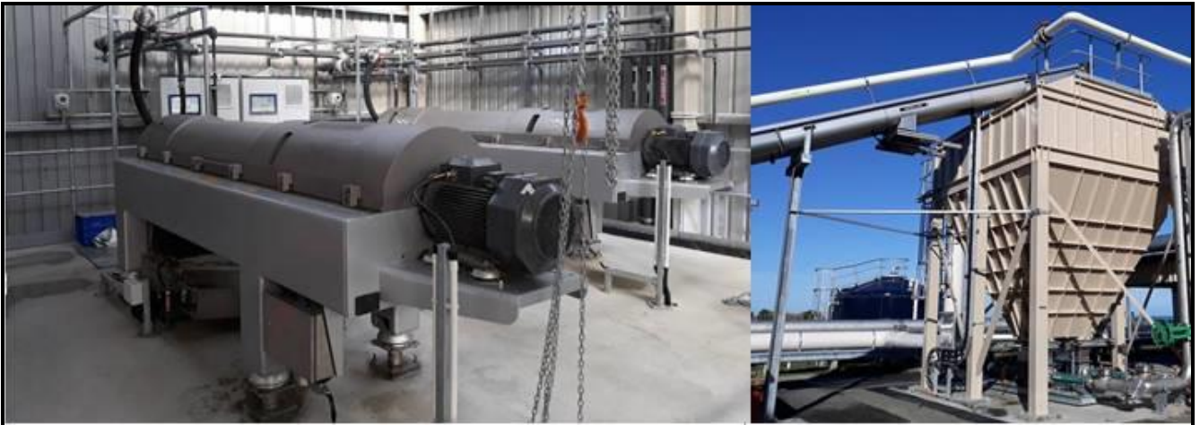
Photograph 13/14: Thermal Sludge Dryer (left), Dried Sludge Storage/Outloading (right)
