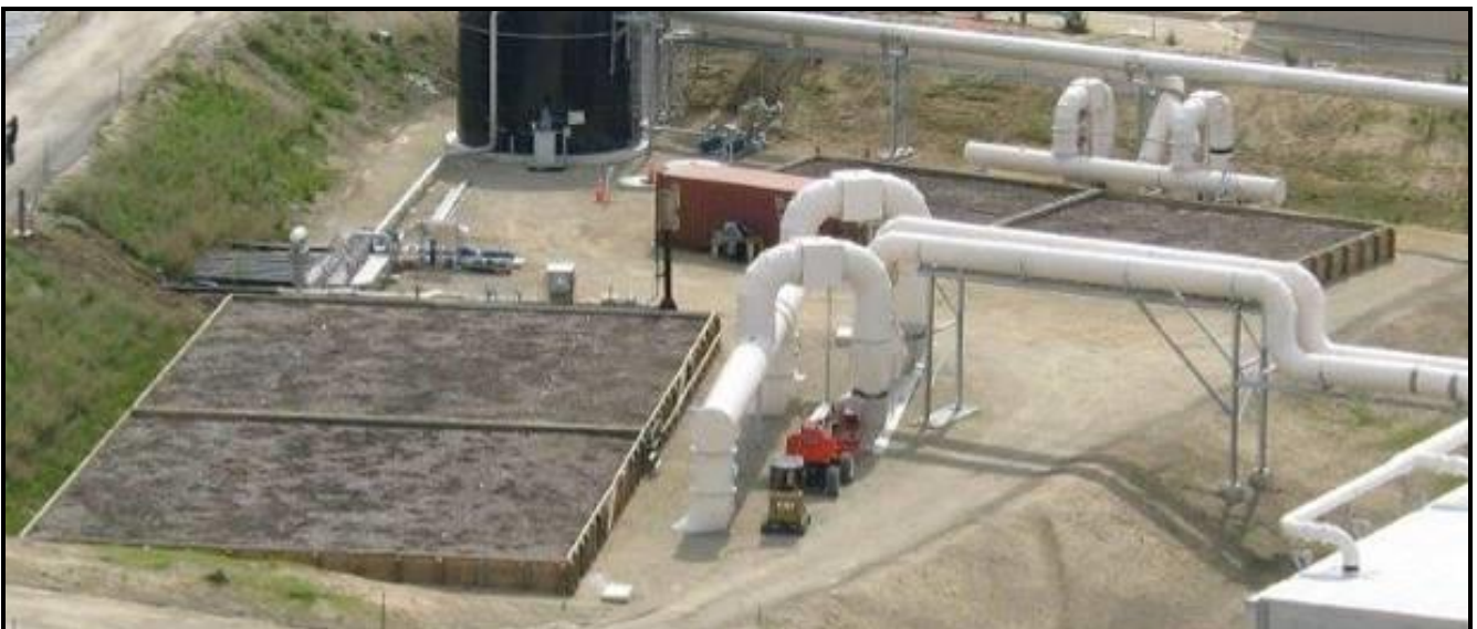
Photograph 16: Biofilters
