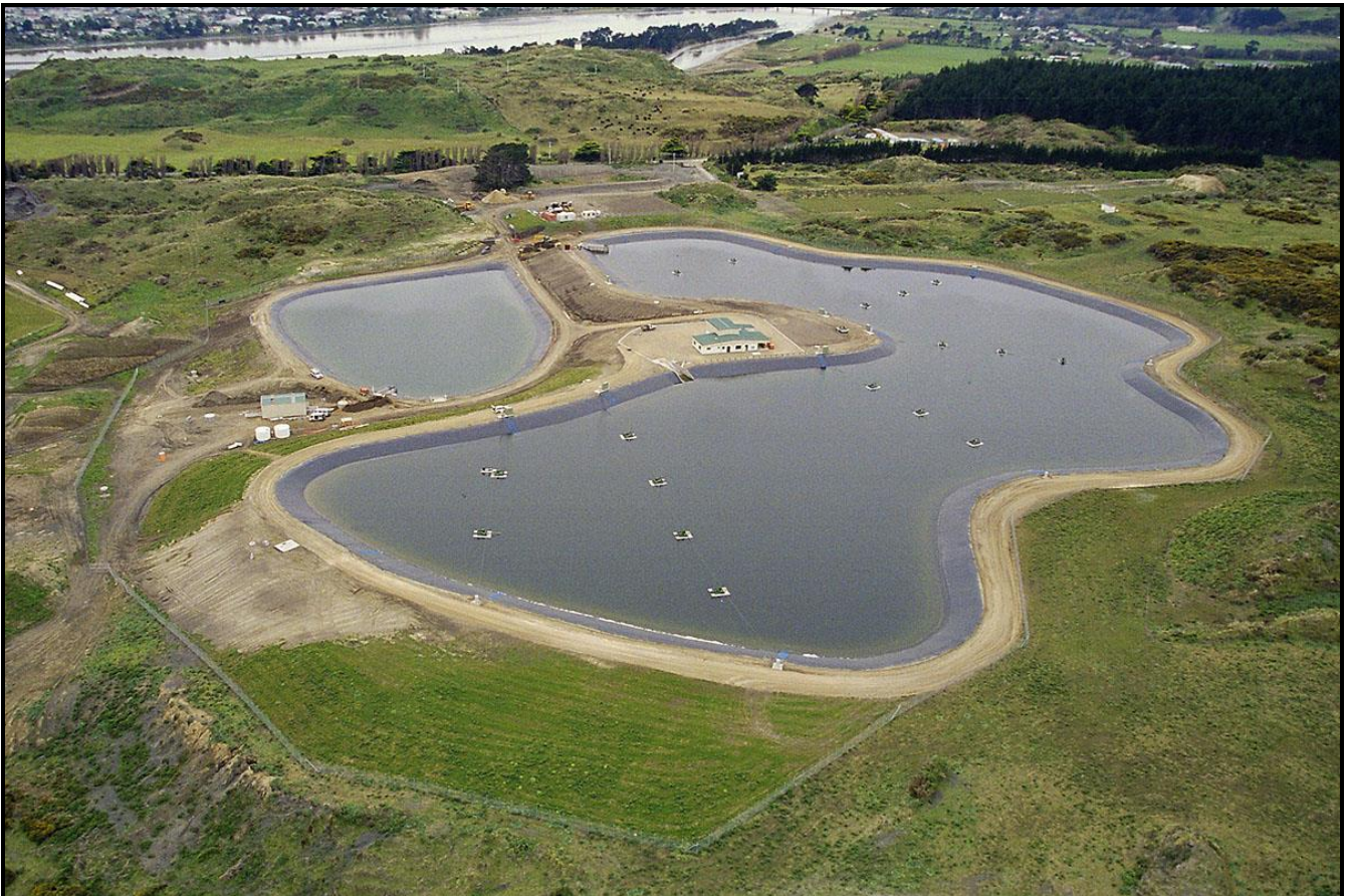
Photograph 1: The Old Wastewater Treatment Plant
