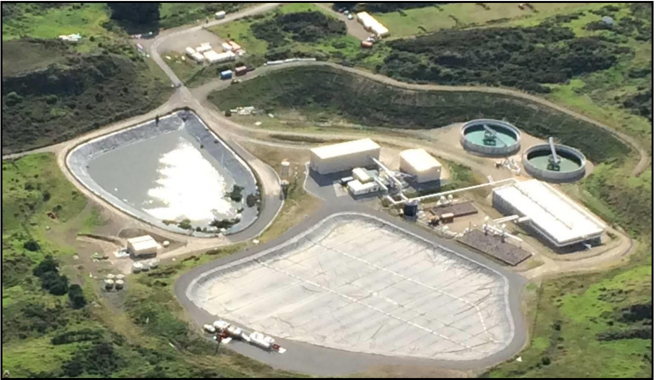
Photograph 2: Aerial View of the new WWTP
